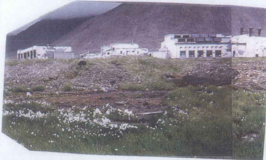
▲ LOOKING S. CULVERT DRAINAGE
