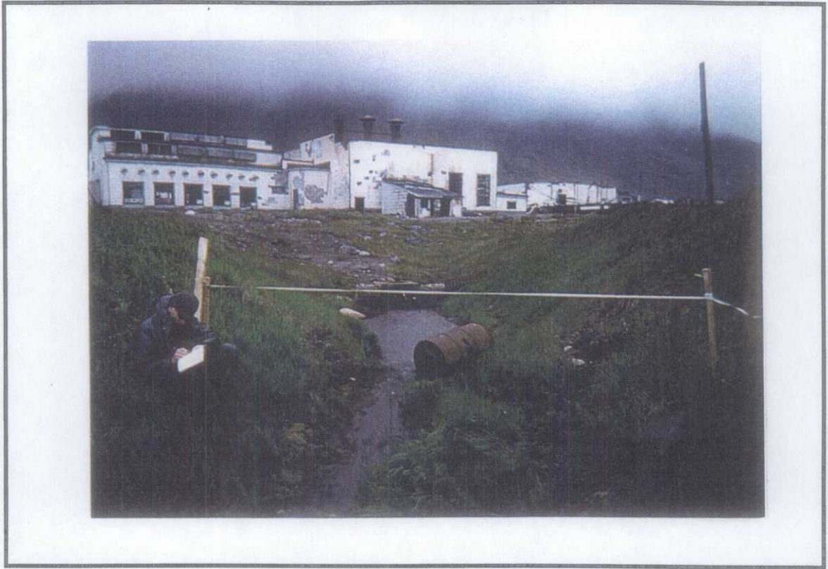
Drainage Basin; view from North, located just North of Site 27. Stream Flow measurement #6 Note empty 55 gal. drum, manhole in center. Site 13 in background
