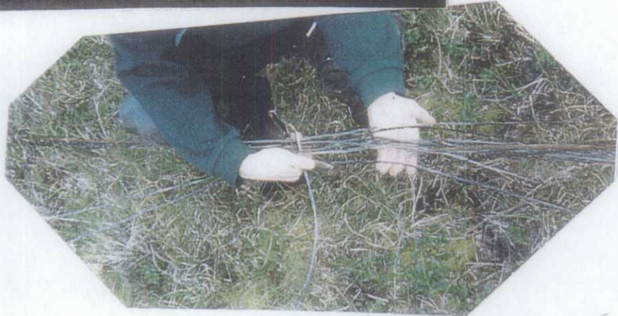
MULTI-STRAND GROUNDED COPPER WIRE
