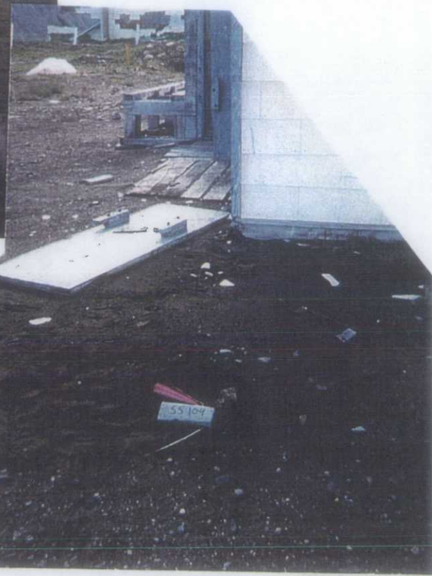
NE CORNER SURFACE SOIL SAMPLE ↑
