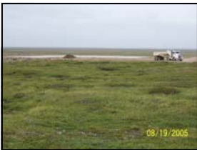
Building 98 Emergency Power, concrete pad post demolition (2005)
