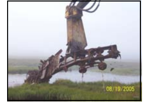
Debris removal at Site 9 (2005)
