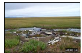
Site 25 prior to demolition (2001)
