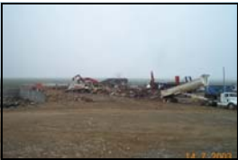
Demolition in progress at Main Complex (2003)
