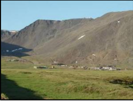
View south towards Main Complex, pre-demolition (2003)
