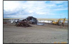
Site 18 - Building 99 under demolition (2003)
