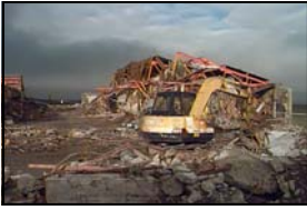
Building 98 Emergency Power during demolition (2001)
