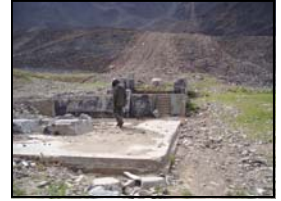
Site 32 Lower Tramway, after demolition and revegetation (2006)
