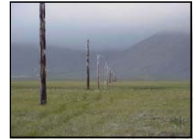
Antenna poles prior to demolition (2001)
