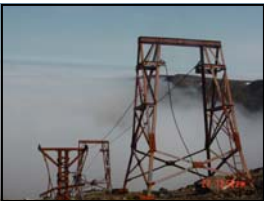
Tram Towers prior to demolition (2005)
