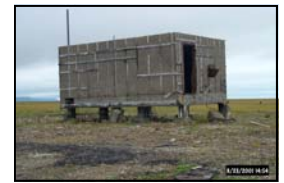
Receiver building prior to demolition (2001)
