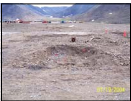
Excavation of PCB-contaminated soils near Site 13 Building 110 (2005)
