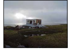
Fuel pumphouse prior to demolition (2002)
