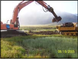
Surface debris removal at Site 9 Landfill (2005)
