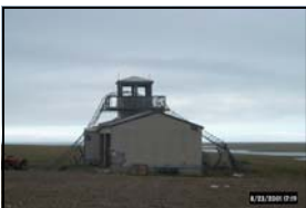
Airport terminal building prior to demolition (2001)
