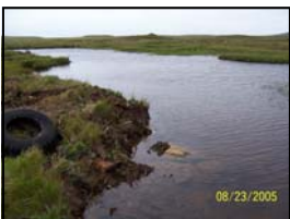
Site 9 Housing and Operations Landfill area, after surface debris removal (2005)
