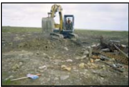
Excavation of test pit at Cargo Beach Road Drum Field (2001)
