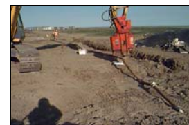
Example of pipeline removal near Main Operations Complex (2001)
