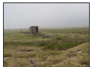
Site 21 wastewater tank prior to demolition (2001)
