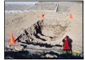
Excavation of PCB-contaminated soils at White Alice site (2005)
