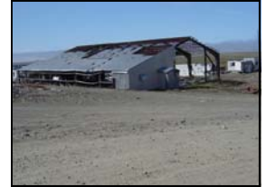
Site 18 - Building 99 prior to demolition (2003)
