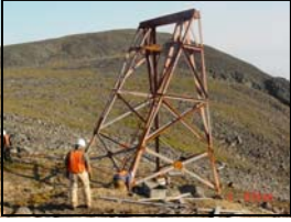
Tramway tower during demolition (2005)
