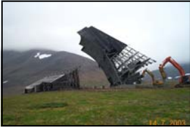
Demolition of White Alice antennas (2003)
