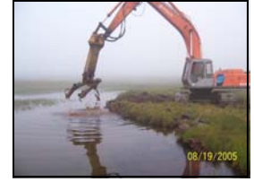
Debris removal at Site 9 (2005)
