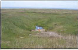
Site 28 Drainage Basin, western culvert (2006)
