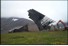
Demolition of White Alice antennas (2003)
