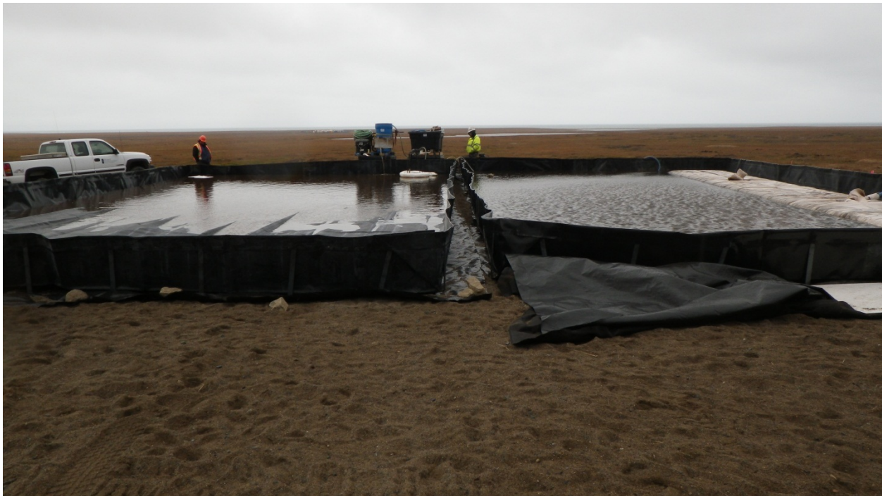
Photo 24 Overview of Containment No. 1 (right) and Containment No. 2 (left) with dewatering geotextile container and water-scrubbing system September 18, 2012
