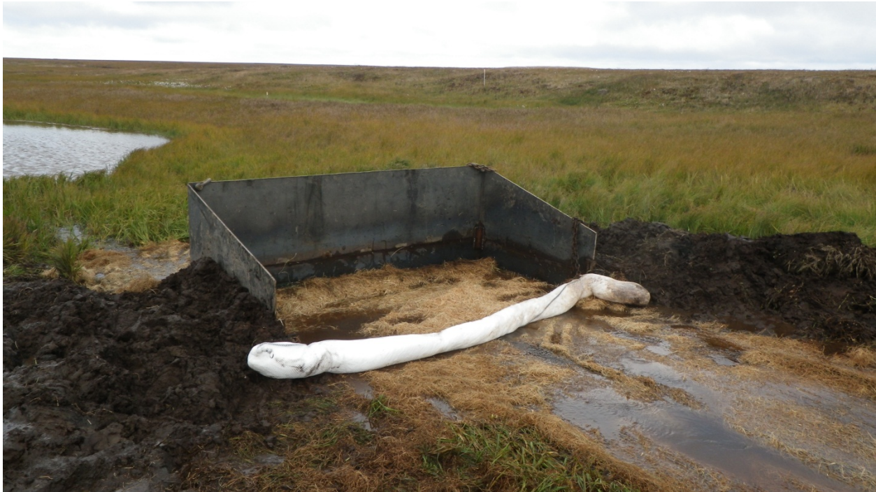
Photograph 11 Sediment trap in place September 15, 2012
