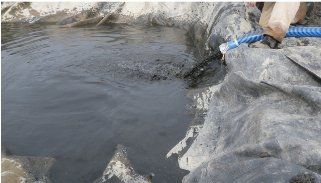
Photograph 18 Sump No. 1 filling directly from dredge September 17, 2012
