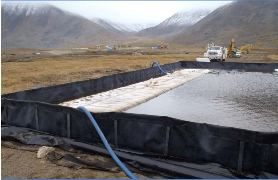
Photograph 21 Containment No. 1 and filling dewatering geotextile container September 18, 2012
