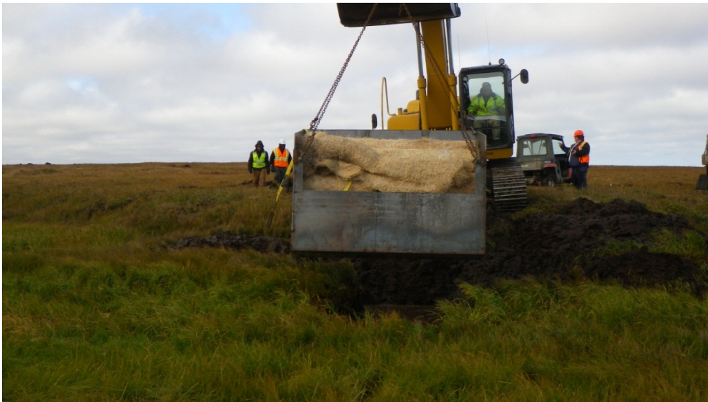
Photograph 10 North of Removal Area 3, sediment trap placement September 15, 2012
