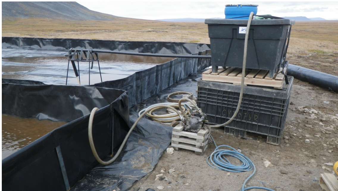
Photograph 22 Containment No. 1 (foreground) and water scrubber Discharging scrubbed water into containment No. 2 (background) September 18, 2012
