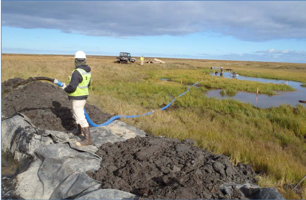
Photograph 17 Dredge effluent discharging to Sump No. 1 September 17, 2012
