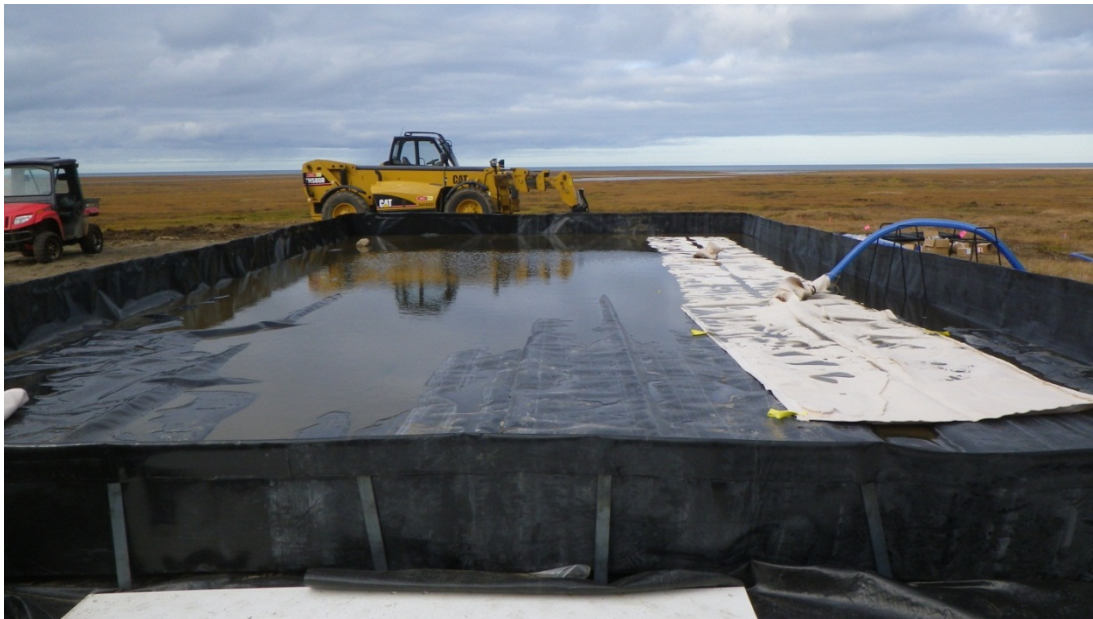
Photograph 20 Containment No. 1 with geotube in place September 17, 2012
