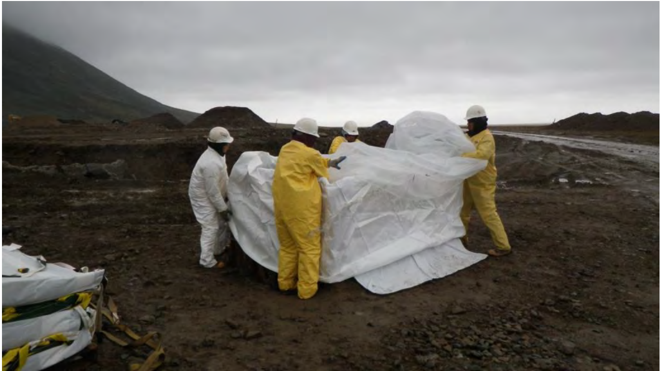
Photograph 51 The bagging crew loads a bag into the frame at the Site 13 PCB excavation. August 19, 2012
