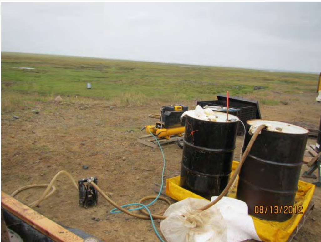
Photograph 46 New bung-top drums were filled with liquid product from drums recovered at Site 10. August 13, 2012
