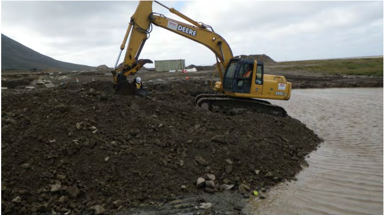
Photograph 53 Backfilling the E-Plume excavation. Floor samples were collected as backfilling progressed. August 24, 2012
