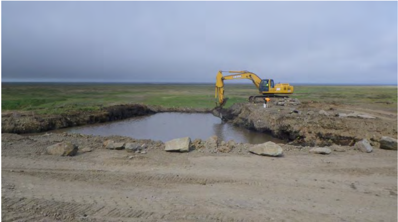
Photograph 47 Collecting field screening samples from the sidewalls of the E-Plume excavation. August 14, 2012
