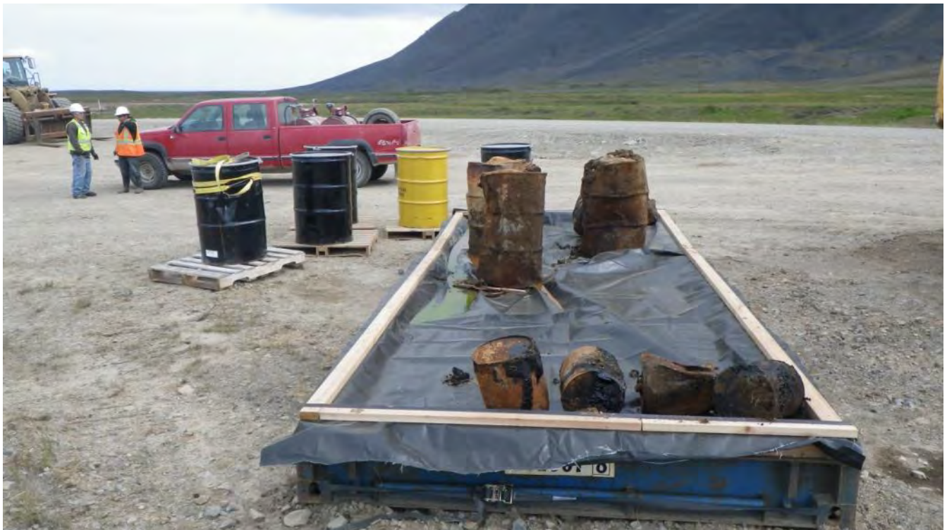
Photograph 42 Over pack drums and the drum containment area. August 10, 2012
