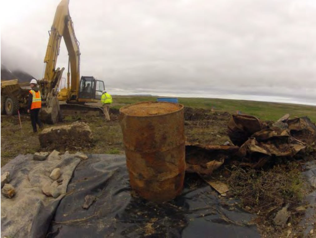
Photograph 33 A drum with unknown liquid removed from the E4 excavation. This drum was placed in an over-pack container. August 2, 2012
