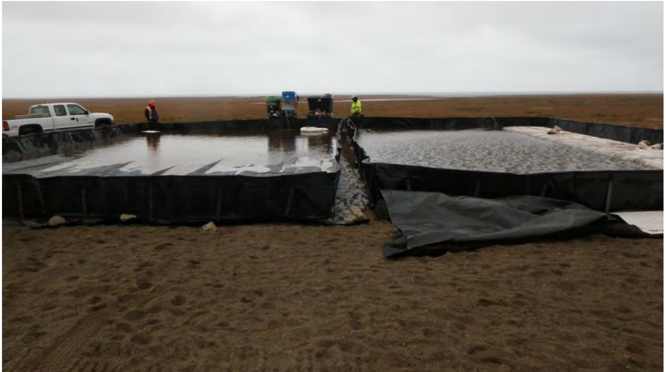
Photograph 77 The primary and secondary impoundments for water dredged from Site 28. September 18, 2012
