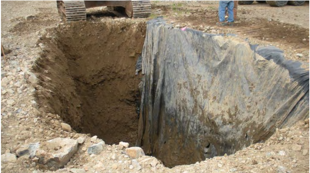
Photograph 19 The curtain liner in the A1 excavation at the MOC. July 21, 2012
