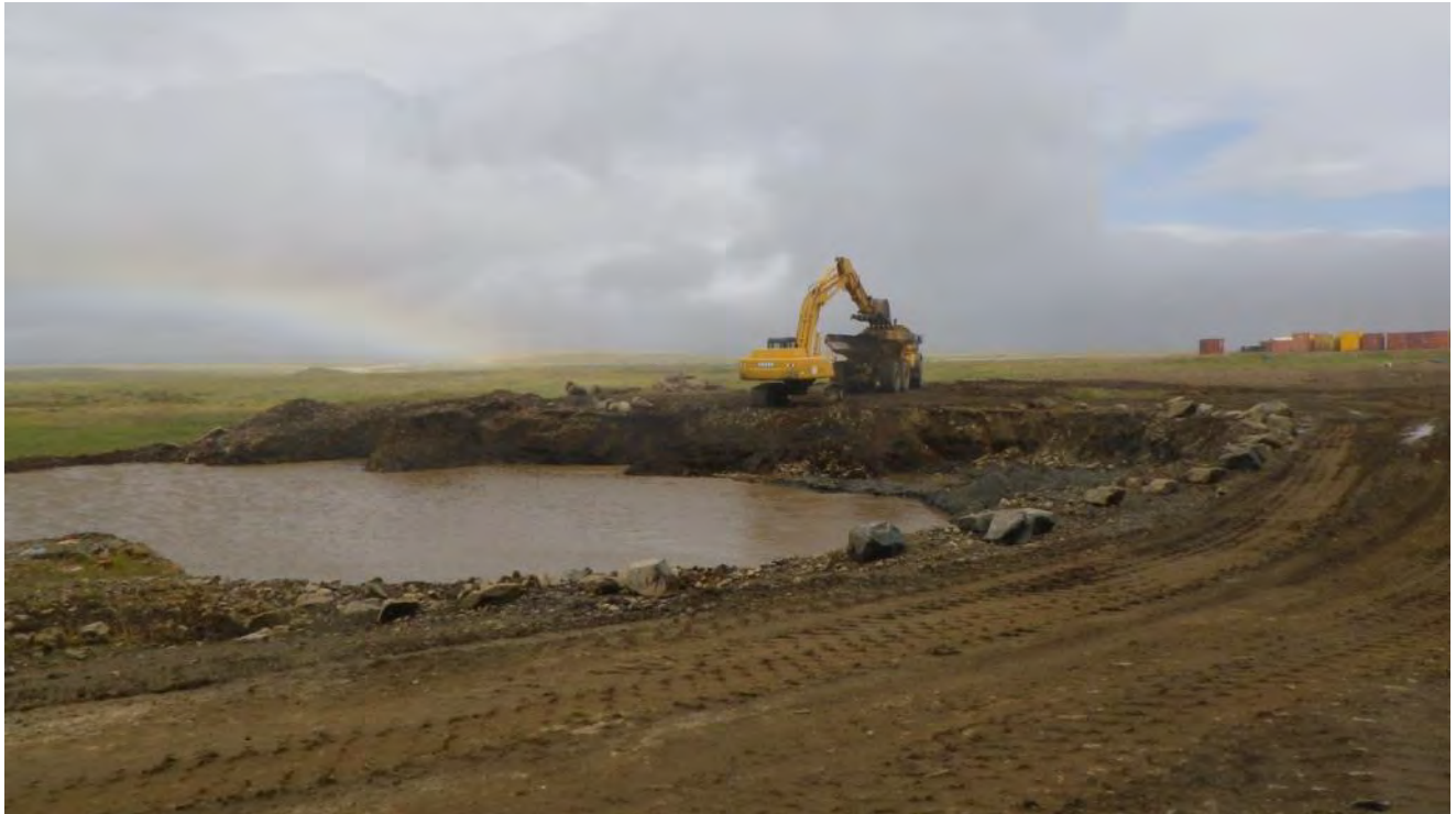
Photograph 49 Excavating contaminated soil at the E plume. August 16, 2012
