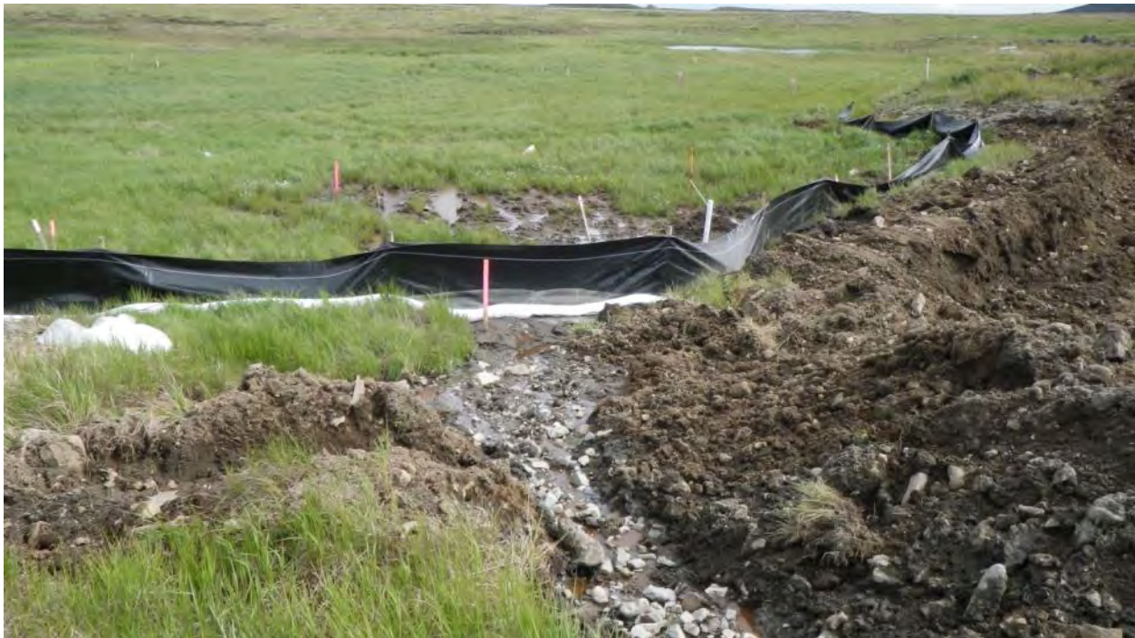
Photograph 34 The Silt Fence and boom at the border between the MOC Pad (near the E Plume) and Site 28. August 3, 2012
