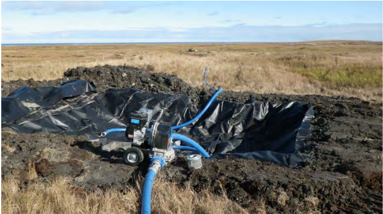
Photograph 75 The secondary impoundment at Site 28 shown with the pump in place. September 17, 2012
