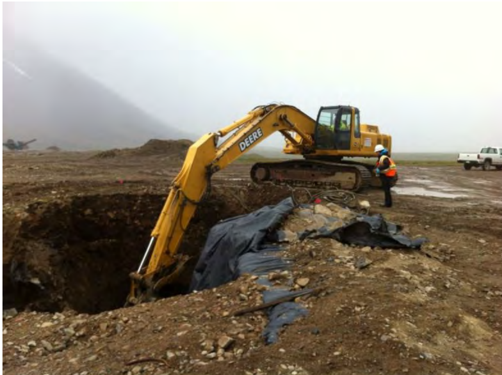
Photograph 24 Excavators were used for sampling deep excavations. Direction: West July 25, 2012
