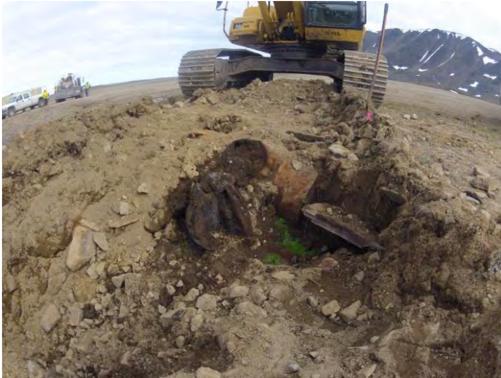
Photograph 9 Antifreeze leaking from exposed drums at Site 10. July 12, 2012
