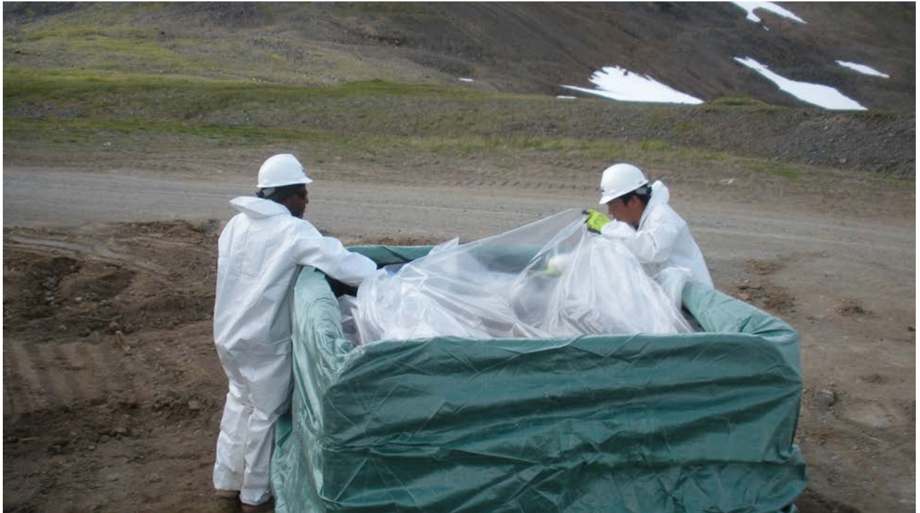
Photograph 13 A bulk bag at Site 31 loaded with soil getting zipped shut in the loading frame. July 14, 2012
