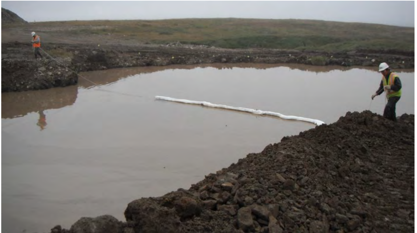
Photograph 55 Boom installed at the E Plume excavation to control petroleum sheen on the surface of the water. August 26, 2012
