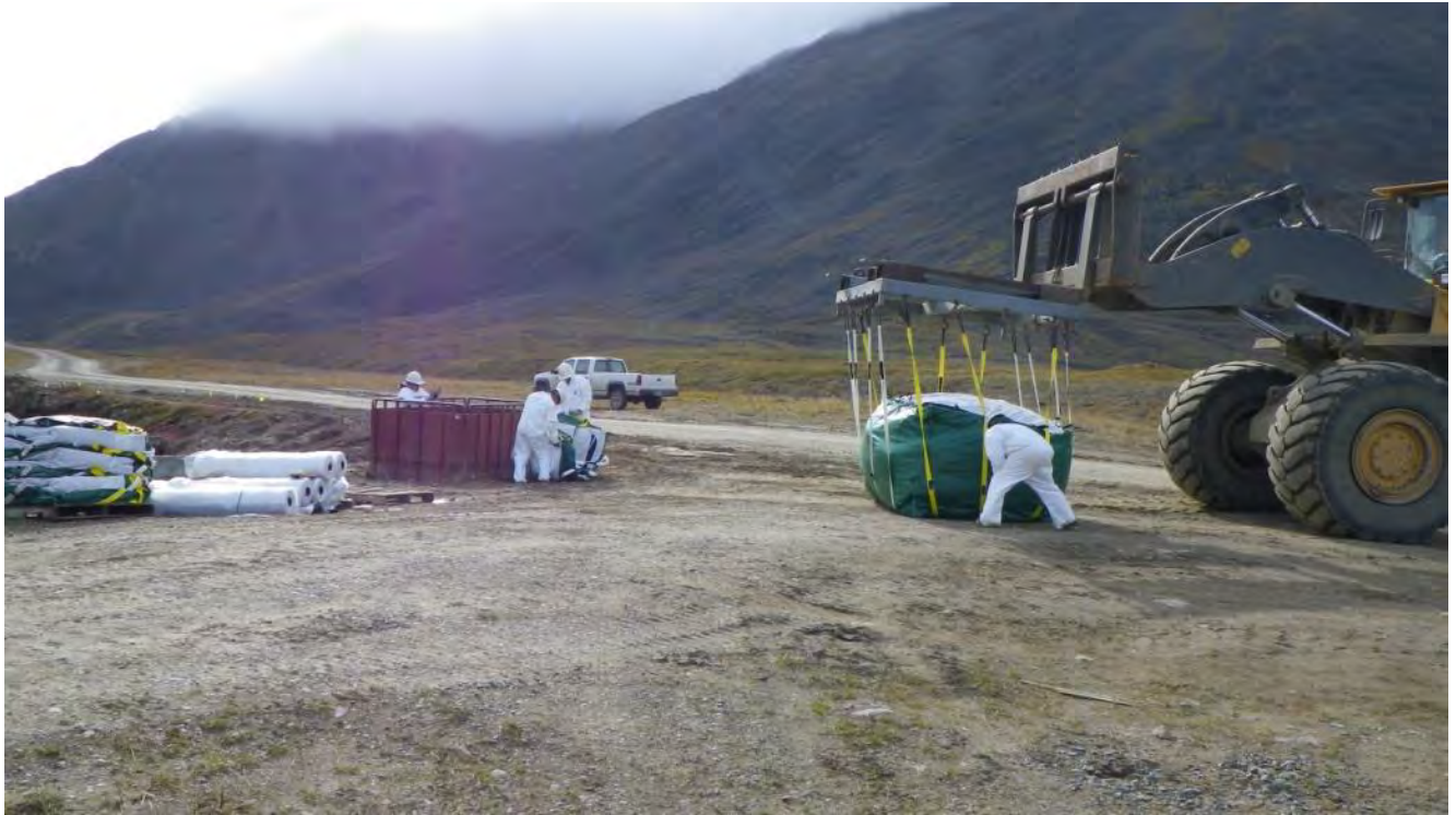
Photograph 69 PCB-contaminated soil excavated from Site 31. Bags are marked for identification. September 11, 2012
