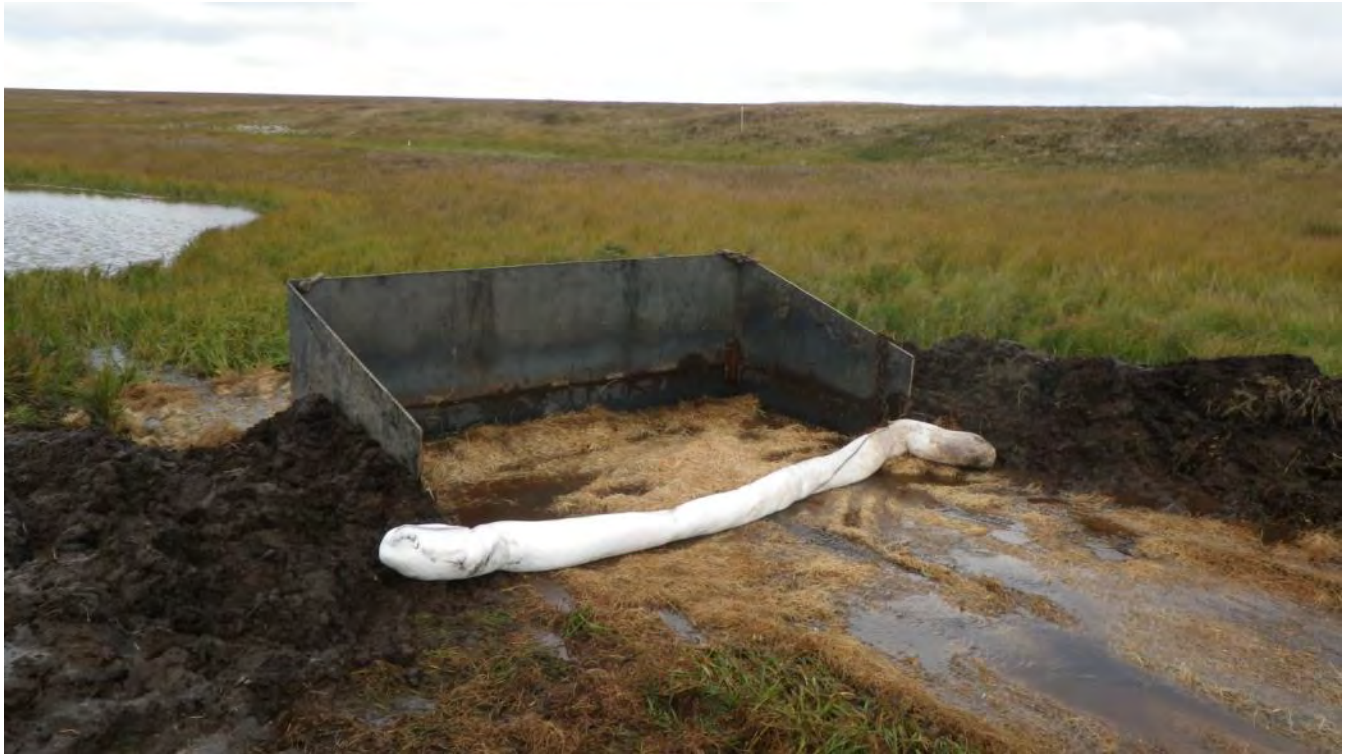
Photograph 73 The sediment trap installed and functional. September 15, 2012
