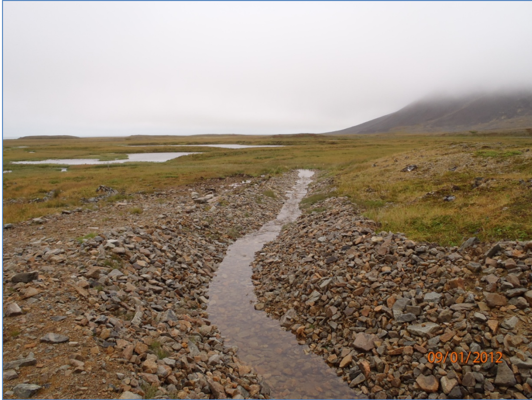
Photo 11: Site 9 Landfill – Diversion ditch in good condition, facing northeast.
