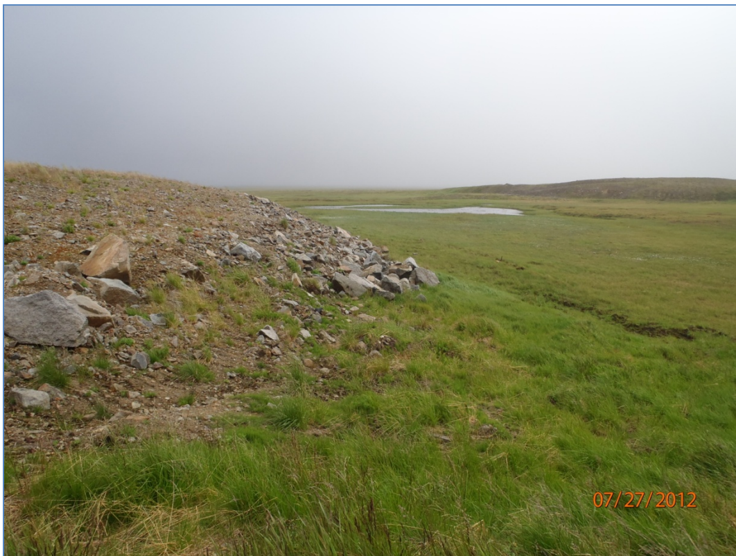
Photo 5: Site 7 Landfill – East side of landfill, facing northeast.
