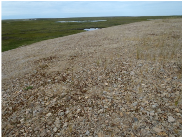
Photo 3: West side of cap, facing NW.
