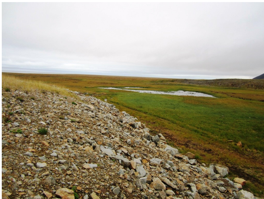
Photo No. 31 – 13 September 2013 Condition of armored rock on the southern border of the landfill cap at Site 7. View facing east.
