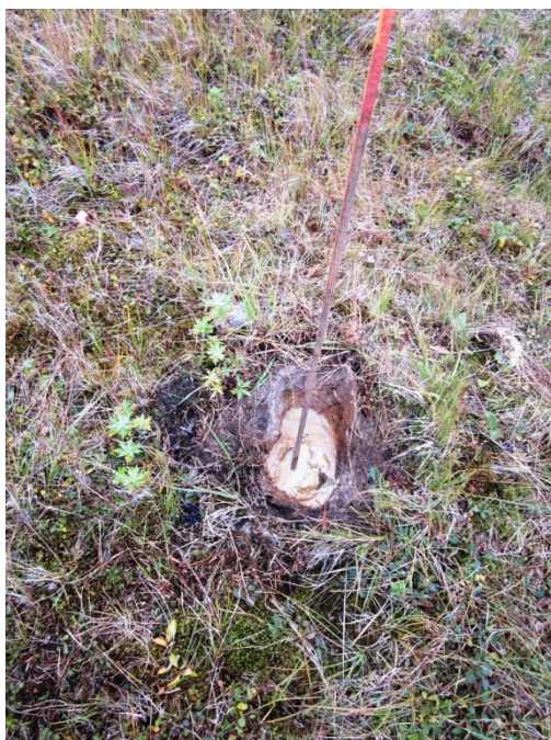
Photo No. 34 – 13 September 2013 Abandoned monitoring well filled with bentonite at Site 7.
