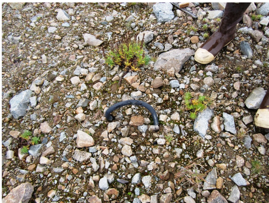
Photo No. 32 – 13 September 2013 Debris protruding through the southern side of the landfill cap at Site 7.
