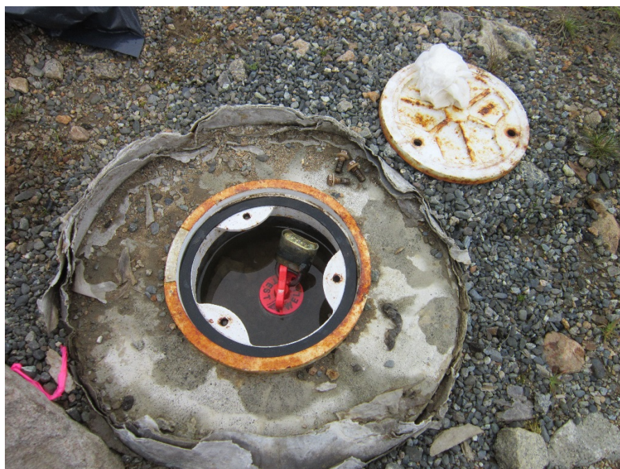
Photo No. 16 – 05 August 2018 Ponded water inside of well casing at flush mount monitoring well 14MW02. View facing down.
