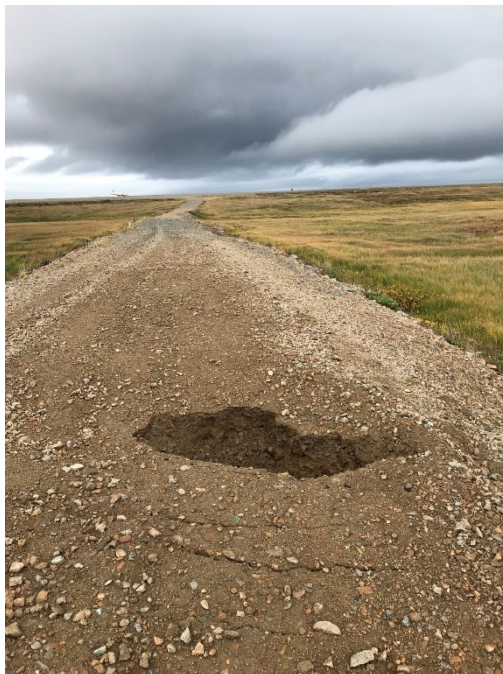
Photo No. 23 – Sinkhole discovered during demobilization site walk along Airport Access Road. View facing northwest.
