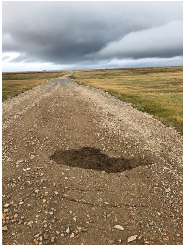
Photograph F-3-2: Sinkhole discovered during demobilization site walk along Airport Access Road. View facing southwest.
