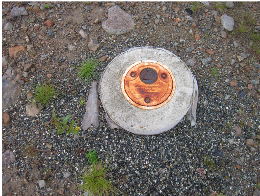
Photo No. 7 – 02 August 2018 View of monitoring well 14MW05. View facing down.
