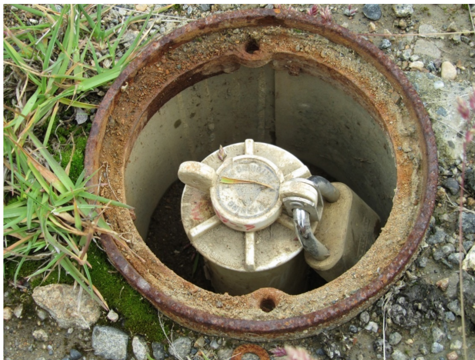
Photo No. 32 – 05 August 2018 View facing down of rusted threads in flush mount at MW88-3.
