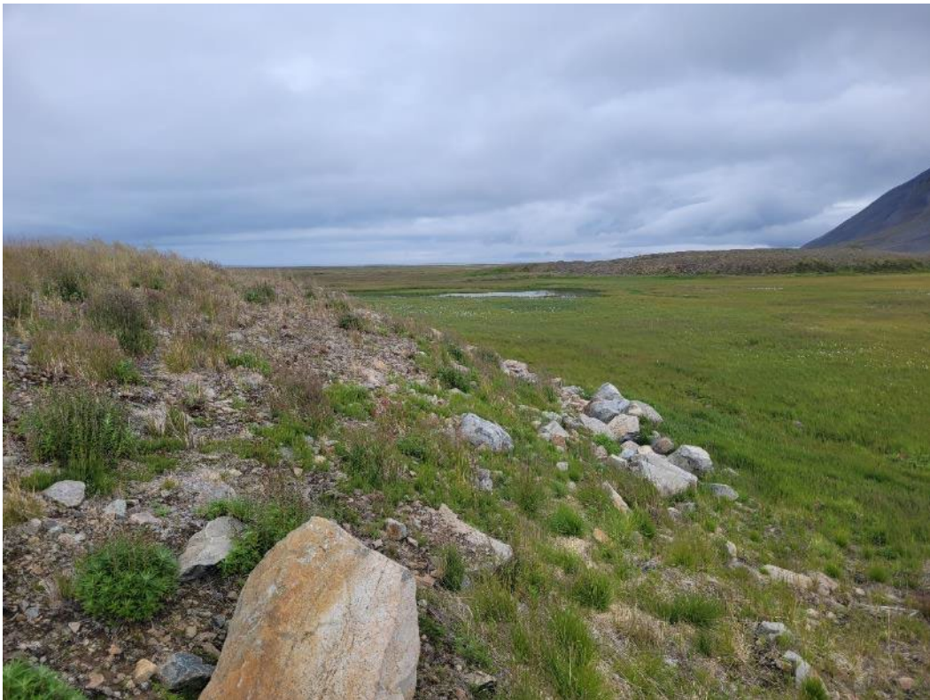
Photo 11: Vegetation growing on lower slope of landfill cap looking SE
