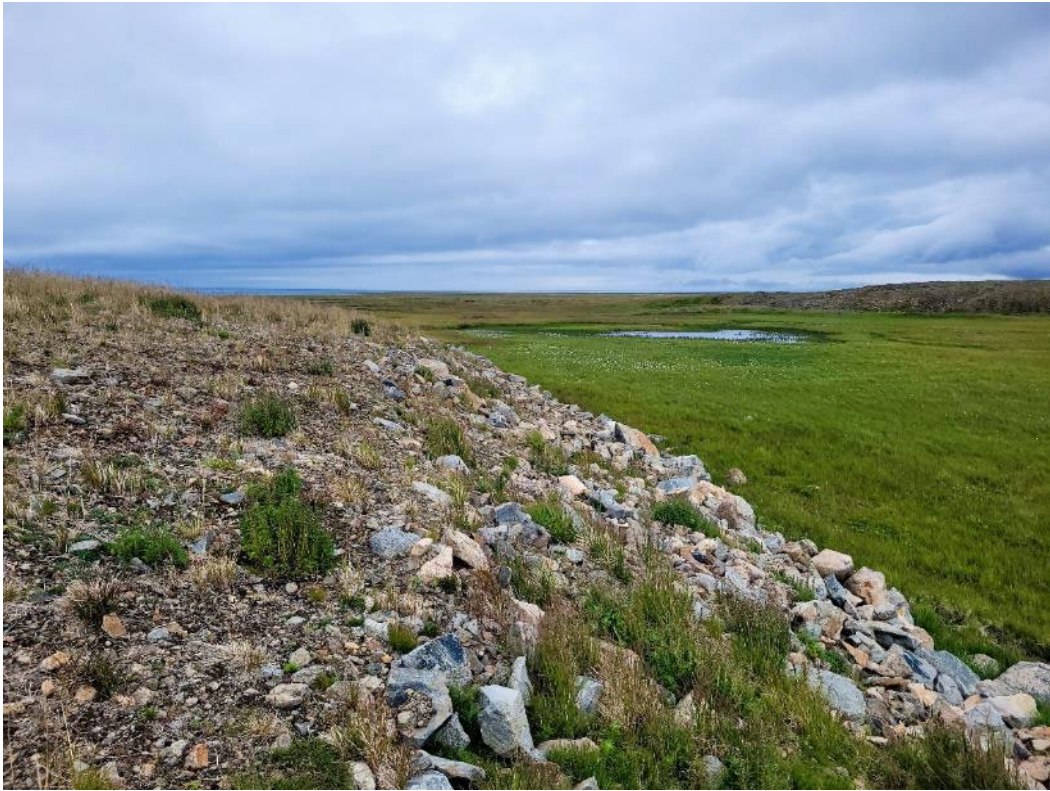
Photo 12: Vegetation growing on lower slope of landfill cap looking SE
