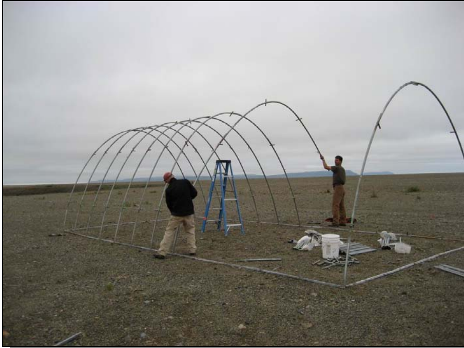
Erecting the Weatherport structure at base camp. (7 August 2007)
