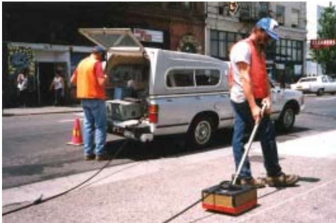
Ground Penetrating Radar
