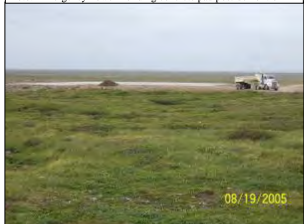
Photo: Emergency Power Building concrete pad post-demolition
