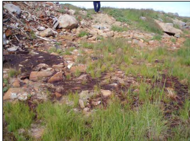
Photo 2. View of petroleum-stained soil at base of eastern portion of Cargo Beach Road Landfill (2006).
