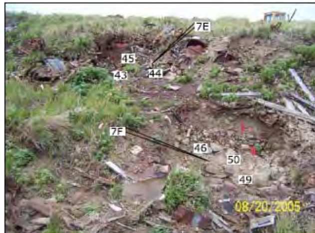
Photo 4. PCB-contaminated soil excavations and confirmation sampling locations (2005).
