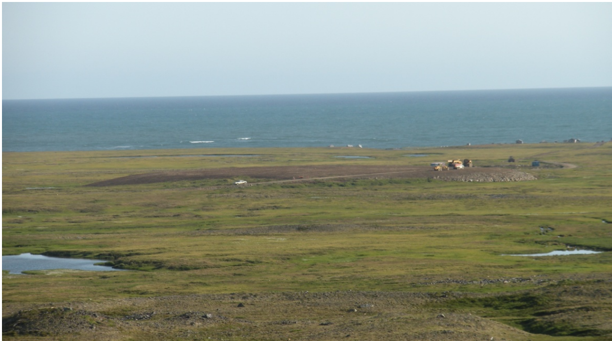
Photograph 8. View looking north at the capped Site 7 Landfill (August 18, 2009).
