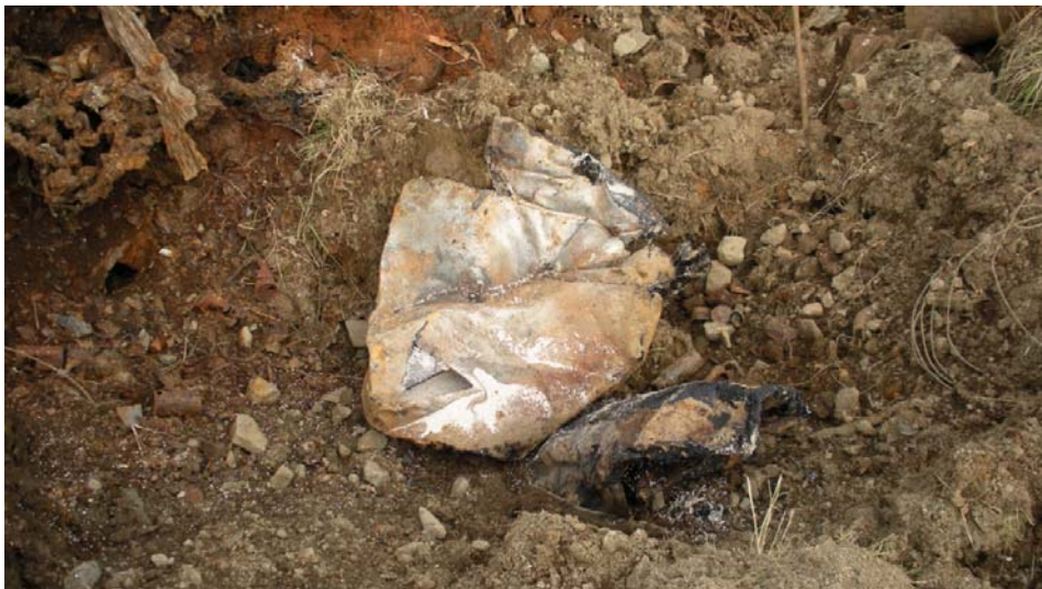
Photograph 4. Crushed drum that was cleaned, coated with Oil-Dri ® absorbent, and returned to landfill.
