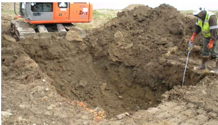
Photograph 1. A 100-square-foot by 4-foot-deep investigation trench in area of metallic anomalies.
