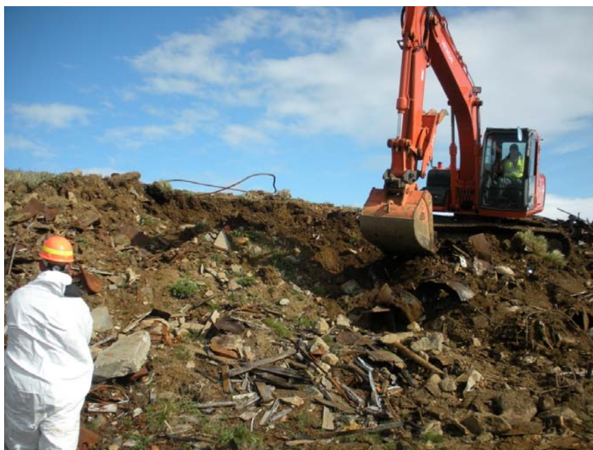
Photograph 2. Excavation of soil and drums from the Site 7 Landfill.
