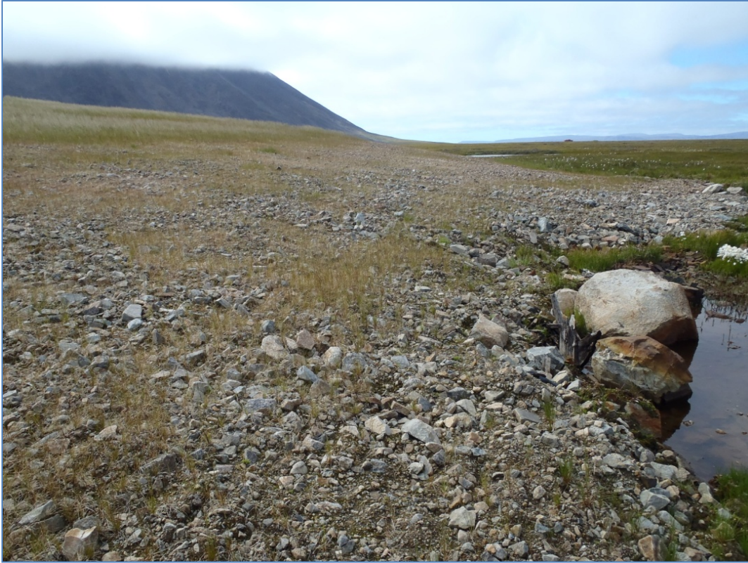
Photo 7: Site 7 Landfill - West slope of landfill, facing south.
