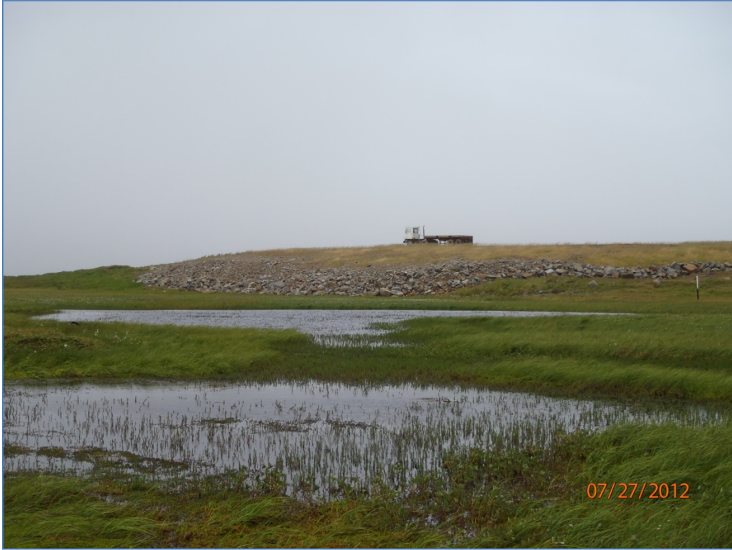
Photo 8: Site 7 Landfill – East side of landfill, facing west.
