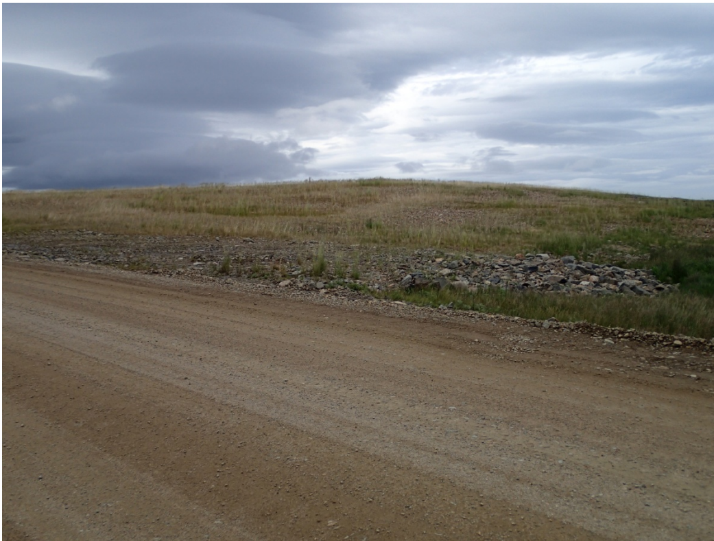
Photo 4: Site 7 Landfill – Southeast side of landfill from Cargo Beach Road, facing NW.
