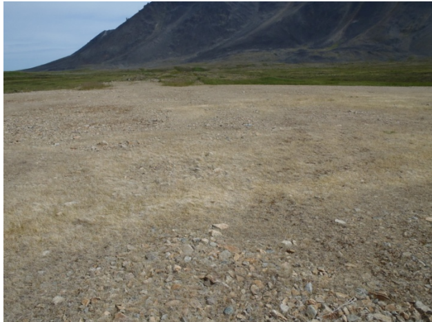
Photo 3: Surface of landfill cap, facing west.
