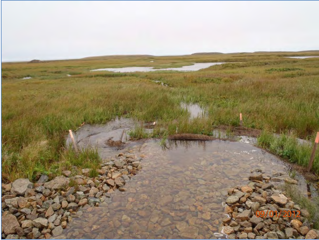
Photo 13: Site 9 Landfill – Diversion ditch outfall area into wetland, facing north.
