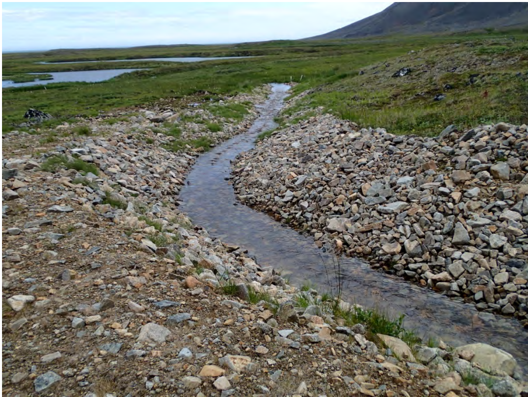
Photo 12: Site 9 Landfill – Diversion ditch that drain pond shown in Photo 11, operating sufficiently, facing NE.
