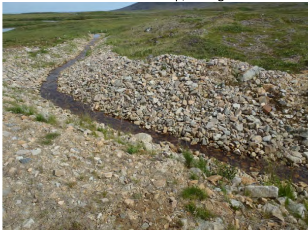
Photo 5: View of diversion ditch, functioning very well, facing NE.
