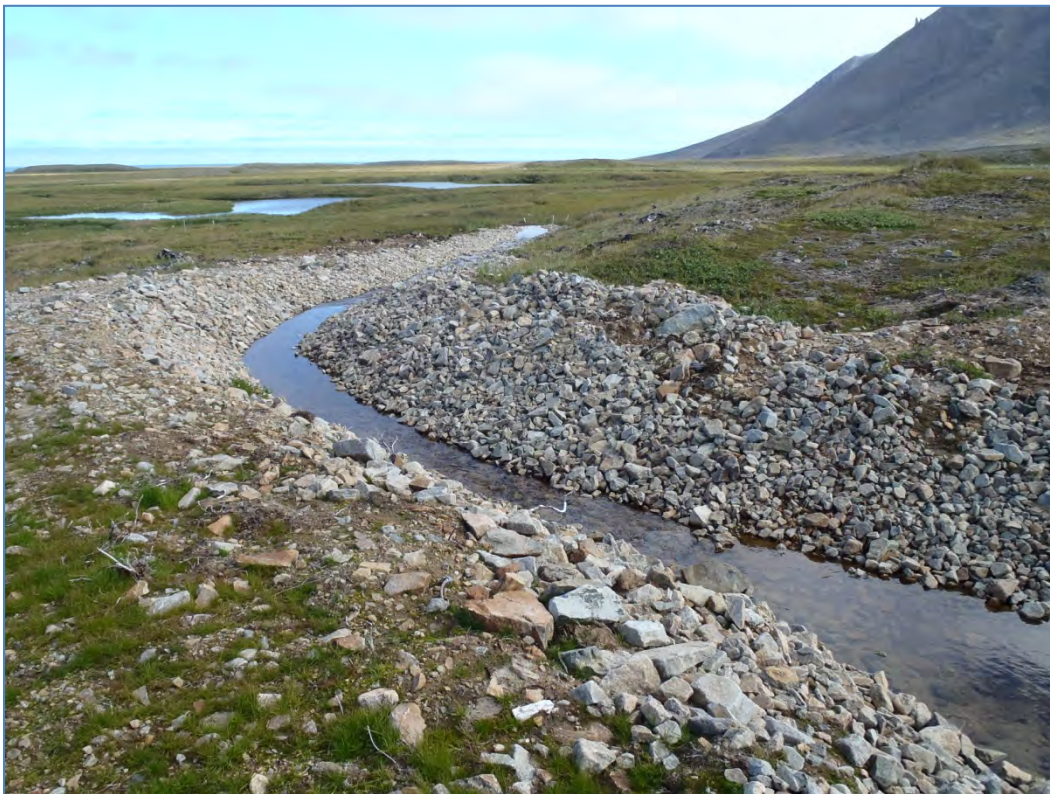
Photo 12: Site 9 Landfill – Drainage ditch operating well and in good condition, facing northeast.
