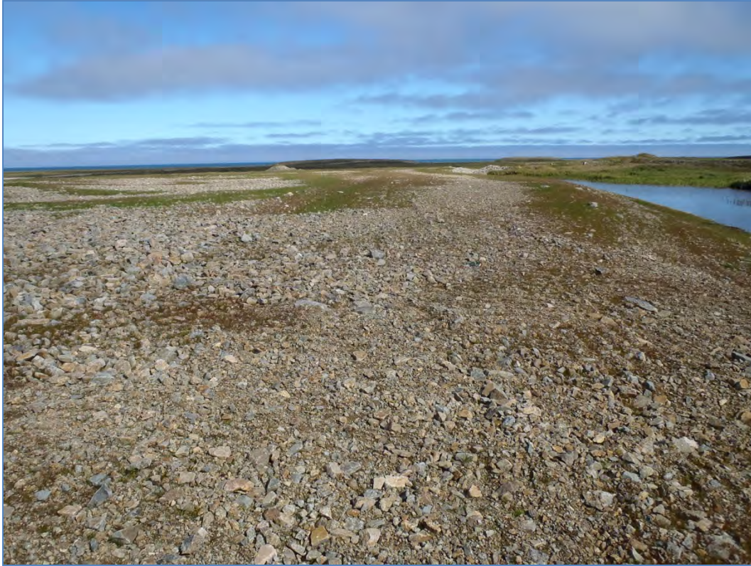
Photo 13: Site 9 Landfill – East side of landfill, facing north.
