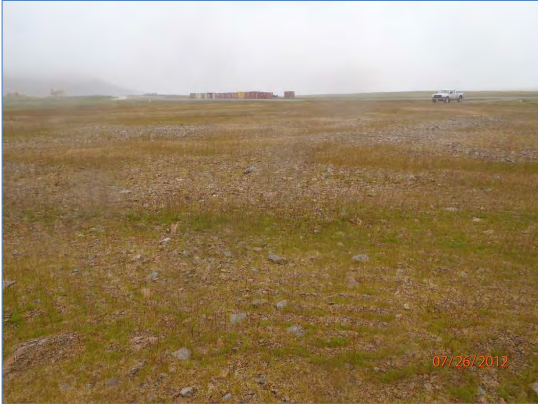
Photo 9: Site 9 Landfill – View of landfill cap surface, facing west with MOC in background.
