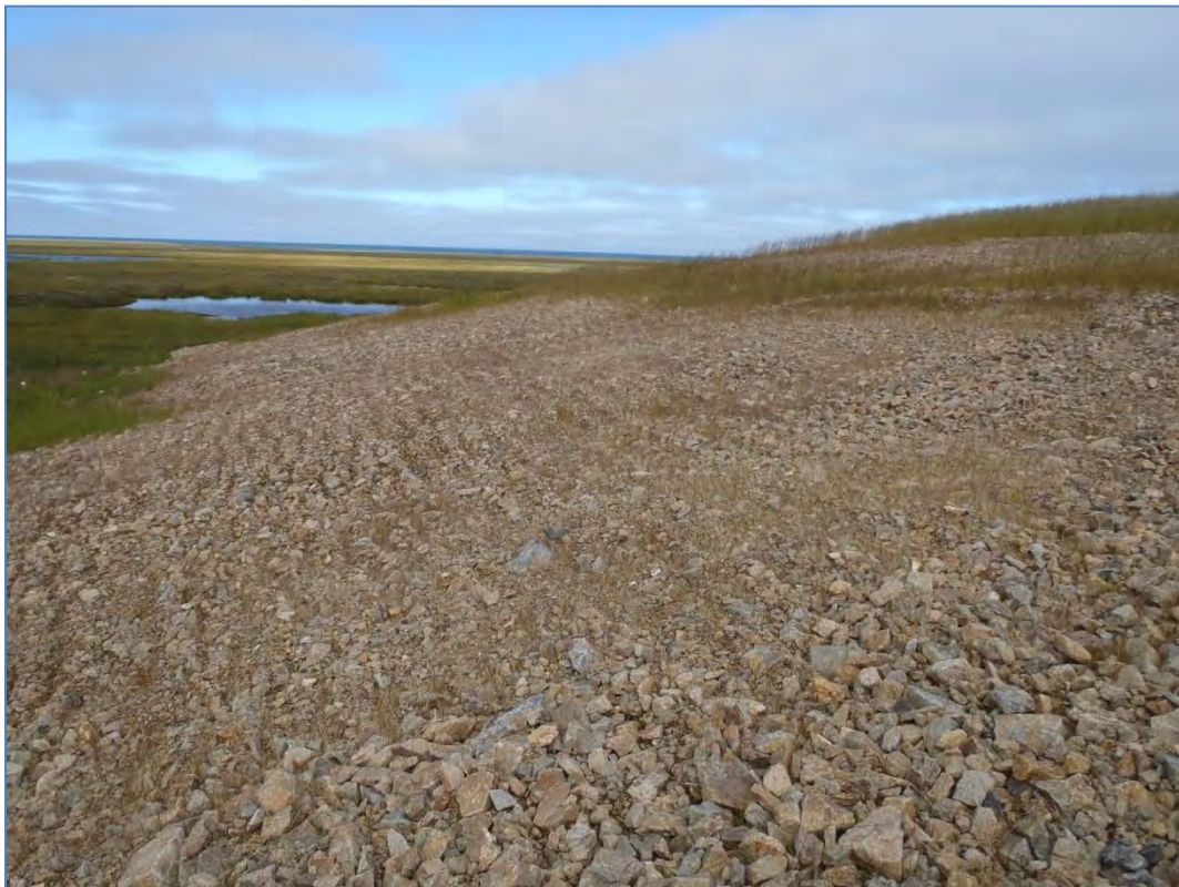
Photo 4: Site 7 Landfill – South slope of landfill, facing west.
