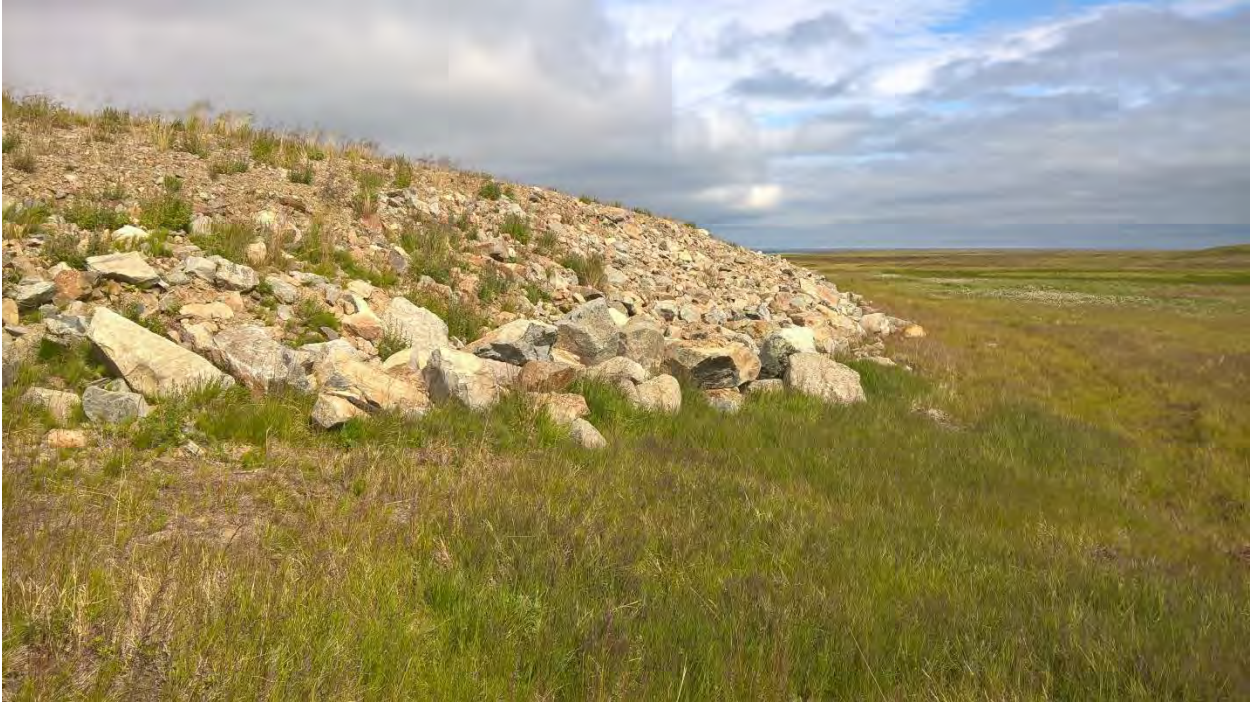
Photo 1: Site 7 Landfill – View of south/southeast slope of landfill with large armor rock and partial vegetation
