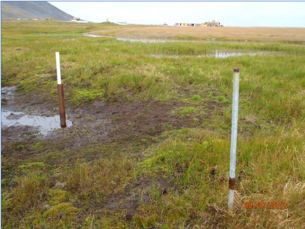
Photo 16: Site 9 Landfill – Drive point well (removed in 2012) and PVC monitoring well on east side of landfill, facing west.
