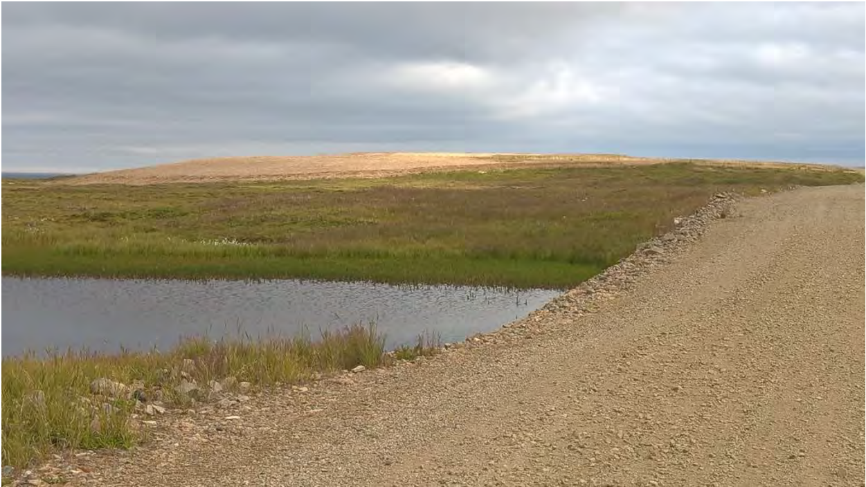
Photo 1: Site 7 Landfill - View of western slope
