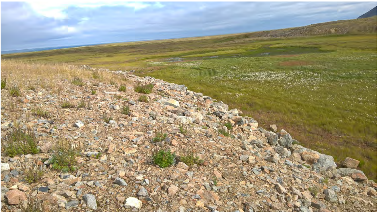
Photo 2: Site 7 Landfill – View of south/southeast slope of landfill with large armor rock and partial vegetation, looking down slope toward tundra
