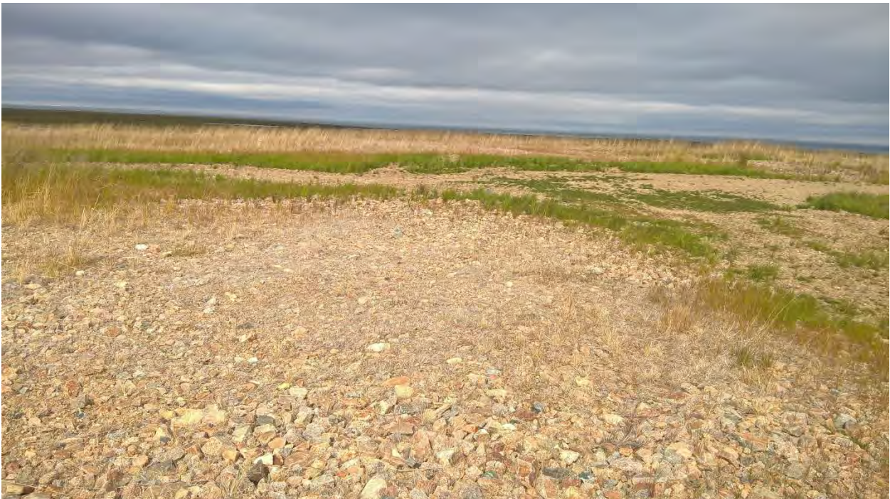
Photo 4: Site 7 Landfill – View looking north, various landfill cap vegetation
