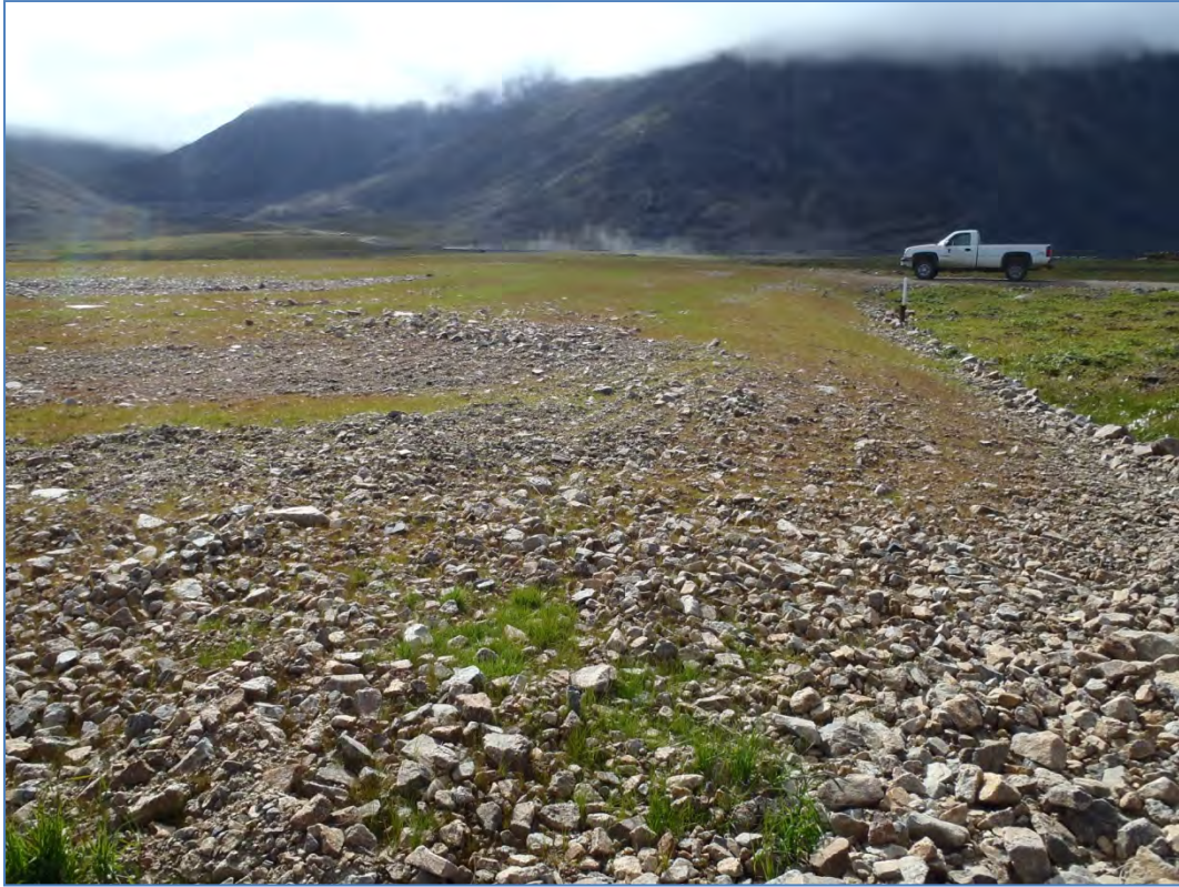
Photo 17: Site 9 Landfill –West side of landfill, facing southwest.
