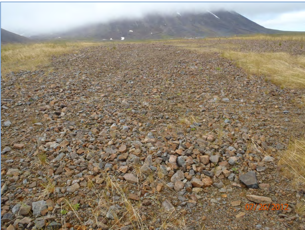
Photo 2: Site 7 Landfill – View of landfill cap from north side, facing southwest.
