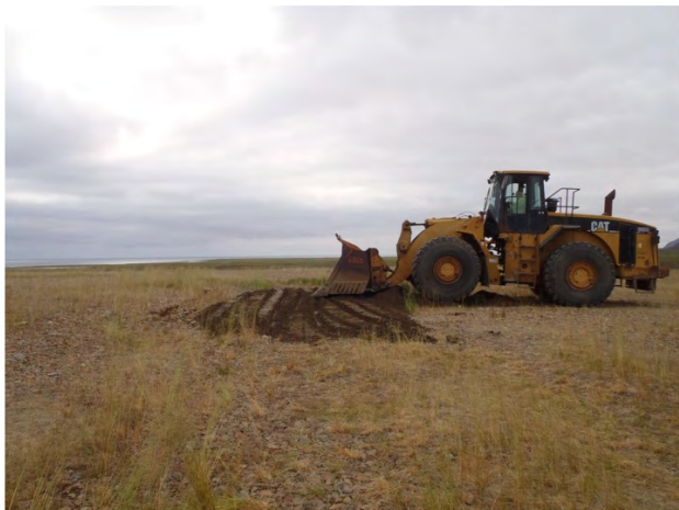
Photo 11: Cap maintenance : A depression near the top of the cap on the west side of the road was filled with clean fine-grained material from the borrow area, compacted, fertilized, and seeded, facing NW.
