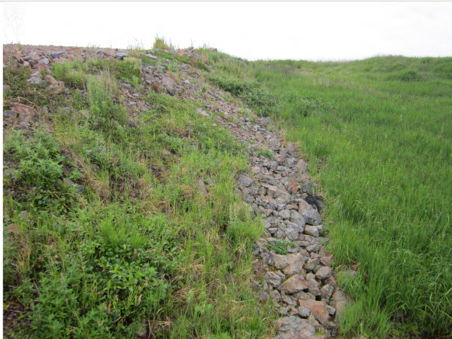
Photo No. 17 – 02 August 2018. Armored rock along the east side of the Site 7 landfill cap. View facing northeast.
