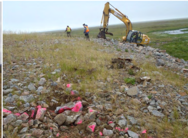
Photo 11: Cap maintenance : A depression near the top of the cap on the west side of the road was filled with clean fine-grained material from the borrow area, compacted, fertilized, and seeded, facing NW.
