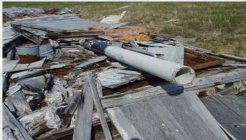
Debris and asbestos transite pipe
