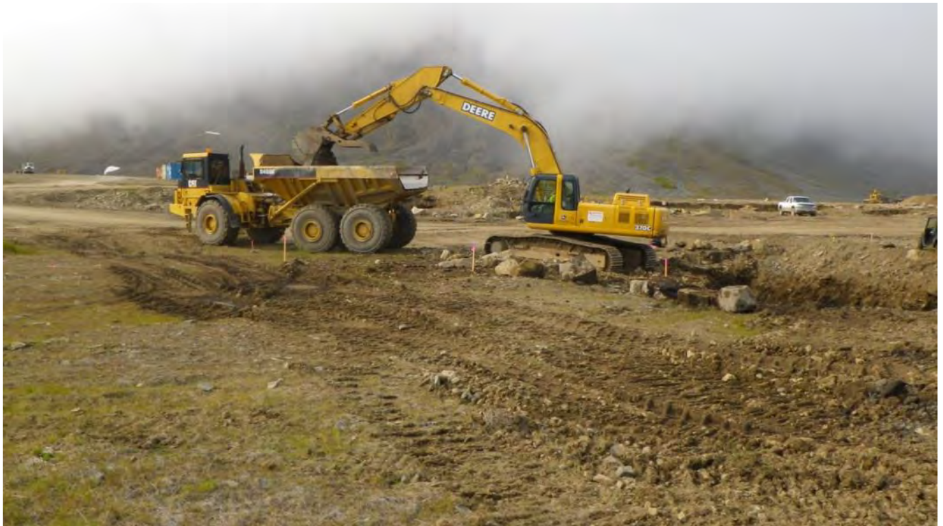
Photograph 36 Excavating at the E3 Plume at the MOC. The tracked excavator is Direction: Southwest loading the rock truck, which will transport the soil to Pad 98. August 5, 2012
