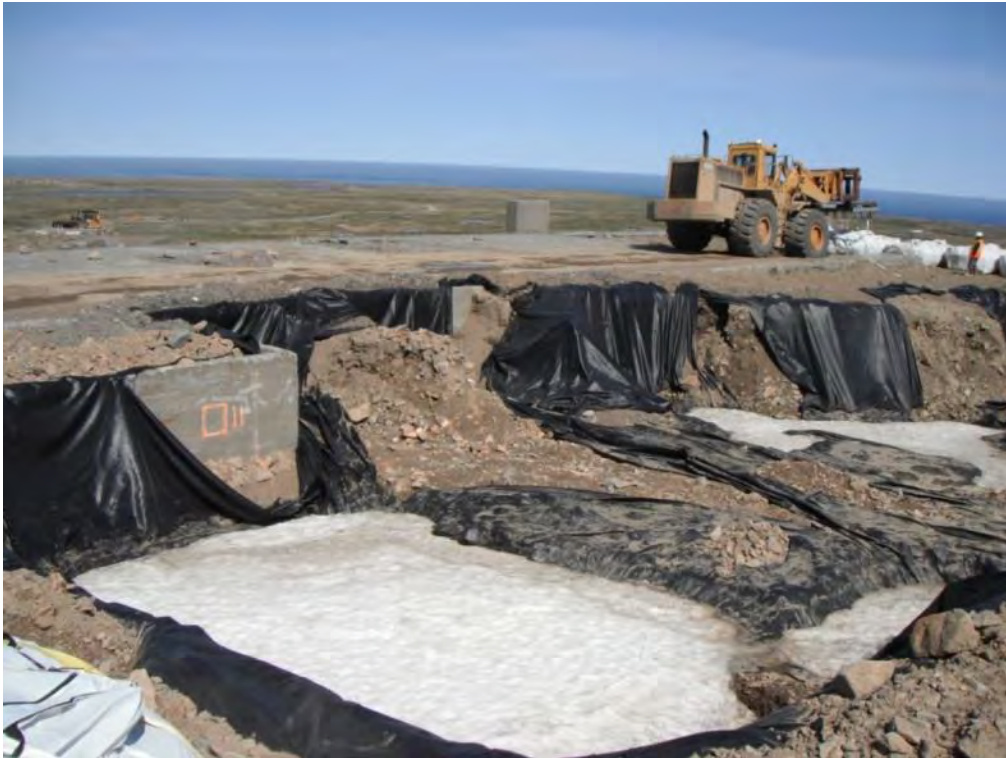
Photograph 3 Liner and overburden being removed from the Site 31 excavation. July 8, 2012
