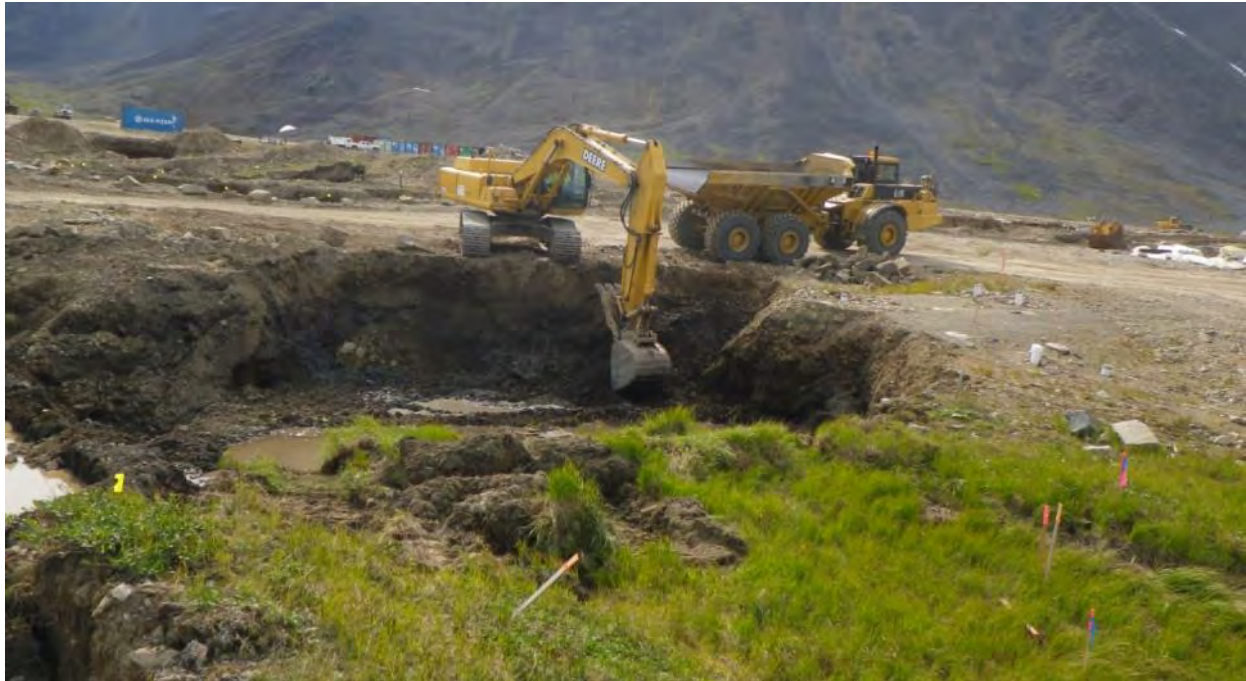
Photograph 41 Excavating POL-contaminated soil at the E3 Plume. August 9, 2012
