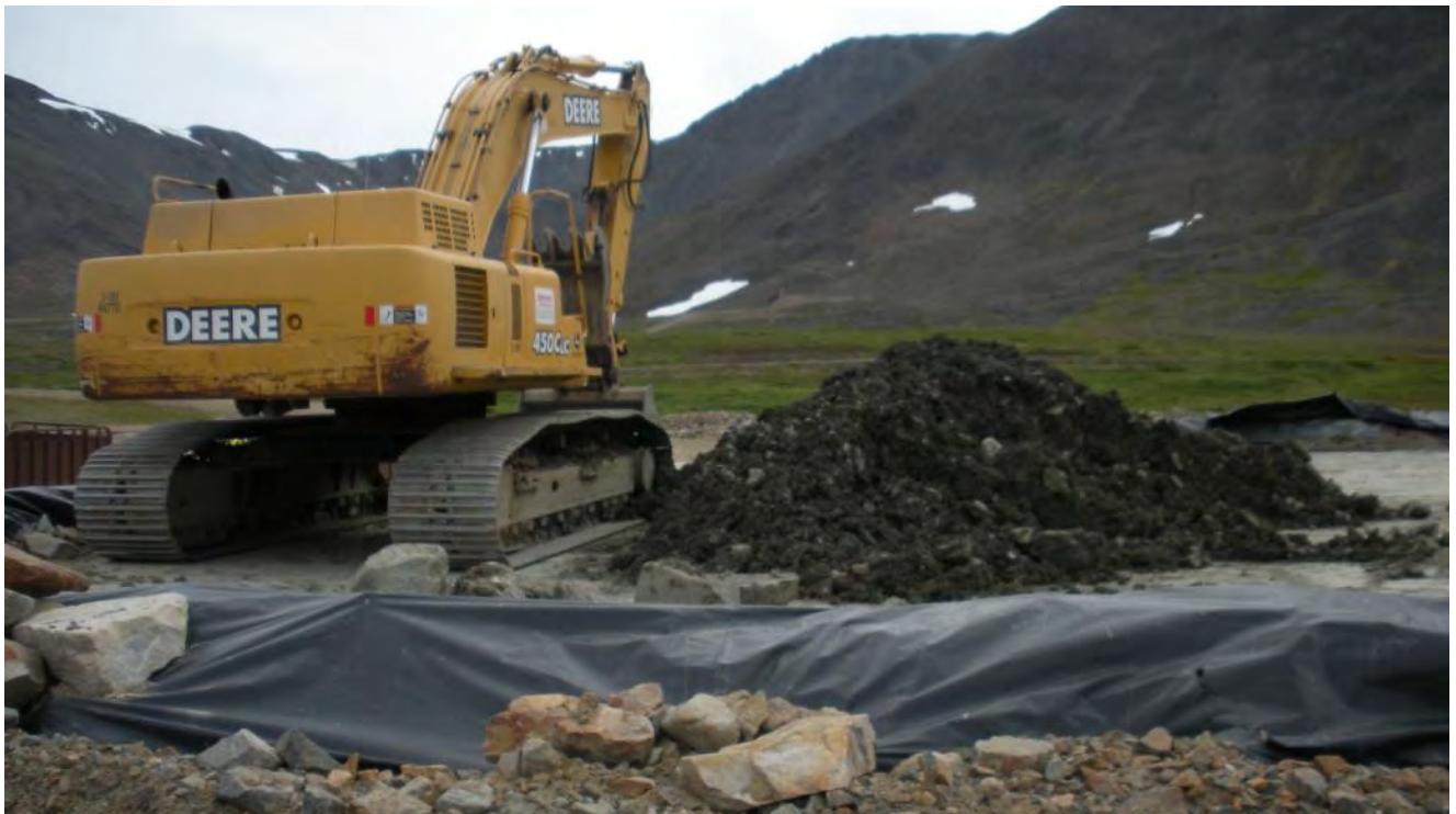
Photograph 22 POL contaminated stockpile at Pad 98. July 23, 2012
