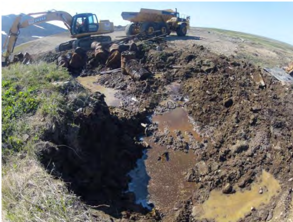
Photograph 8 The excavation at Site 10 with an oil/sheen on the water surface. Direction: Southwest July 11,2012
