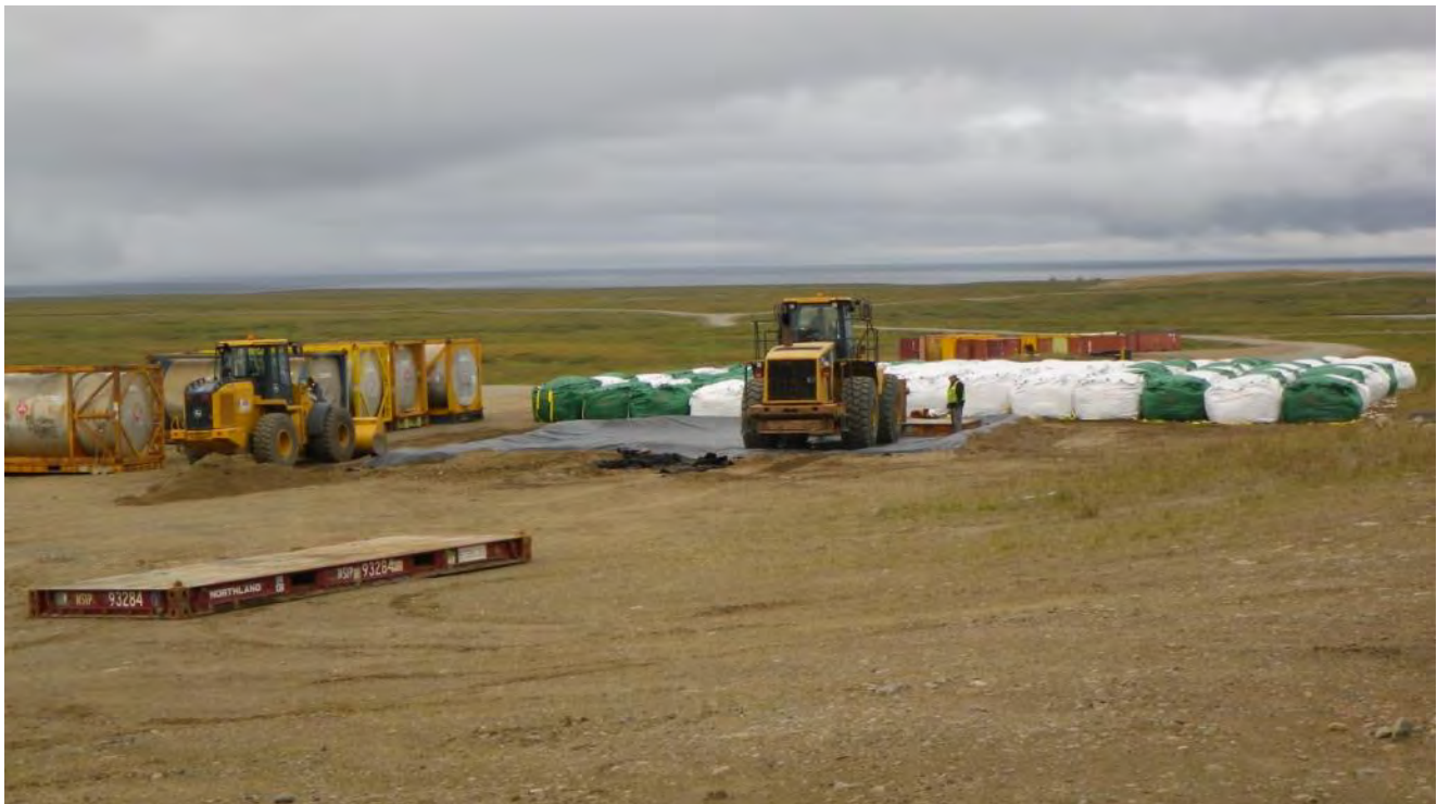
Photograph 50 New liner installed at the fuel containment. August 17, 2012
