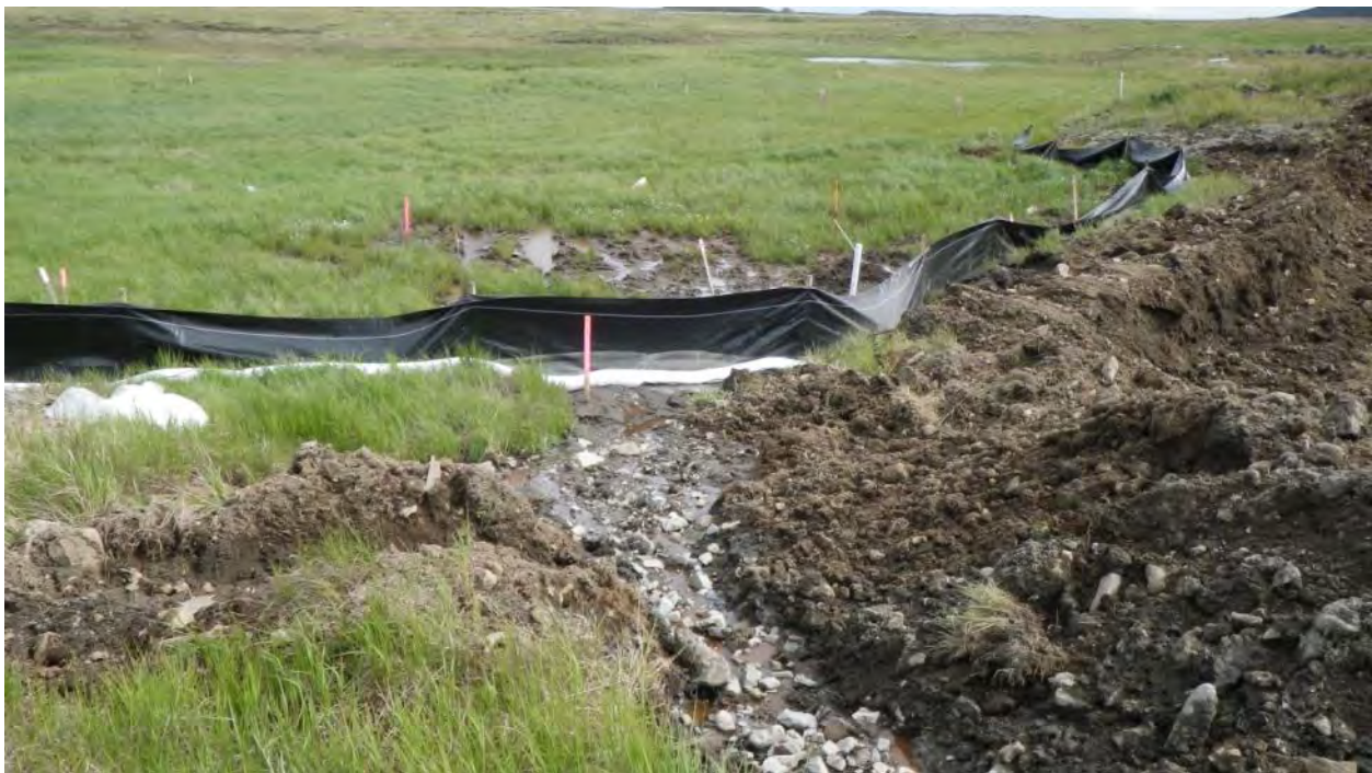
Photograph 34 The Silt Fence and boom at the border between the MOC Pad (near the E Plume) and Site 28. August 3, 2012
