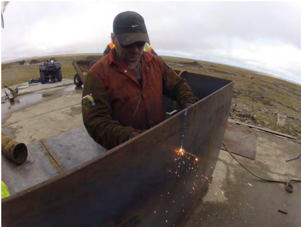
Photograph 66 Construction of the sediment trap that was utilized during Site 28 sediment removal activities. September 7, 2012
