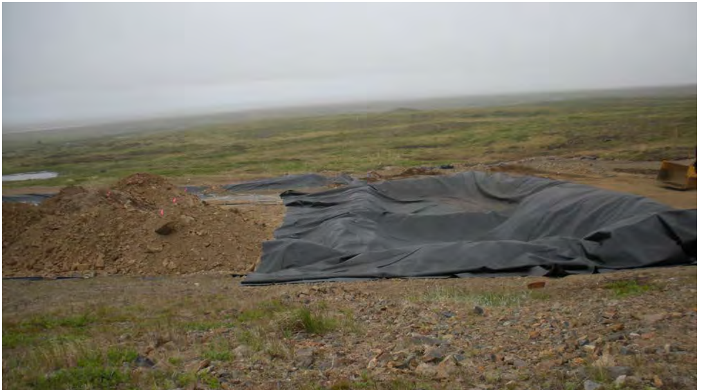
Photograph 12 A lined containment area with bermed sides at the MOC. July 14, 2012
