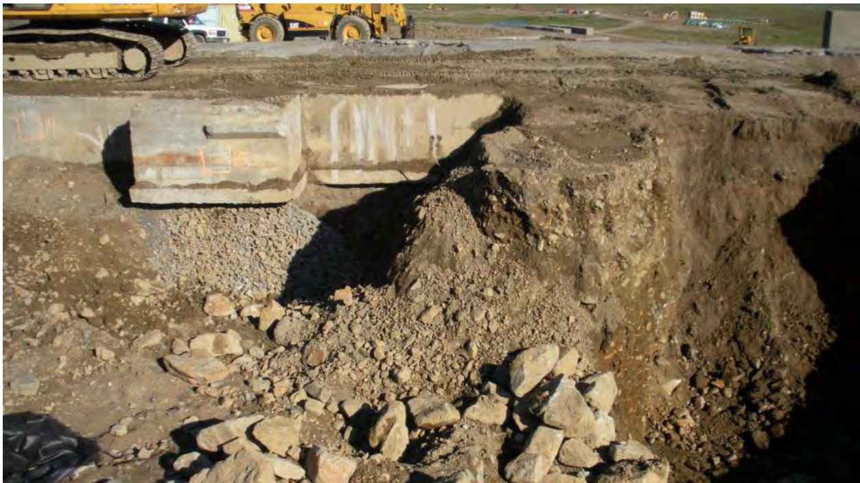
Photograph 30 A concrete sidewall exposed in the Site 31 excavation. Sidewalls were wipe-sampled and submitted for PCB analysis. July 30, 2012
