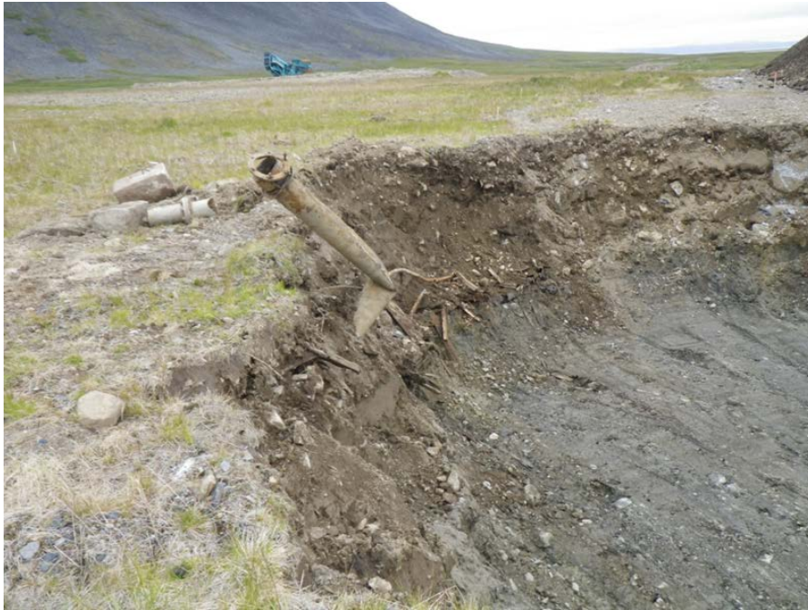
Photograph 17 Buried debris and underground piping Northeast Cape exposed at southern extent of A1 excavation August 6, 2011 Direction: Southwest
