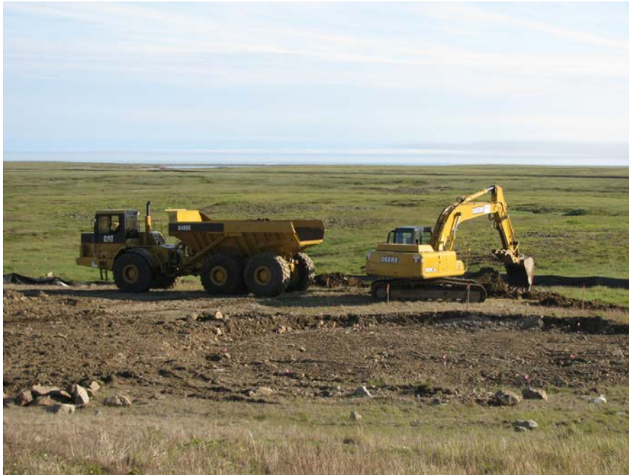
Photograph 13 J1A excavation with silt fence and dump truck for transporting clean overburden July 25, 2011
