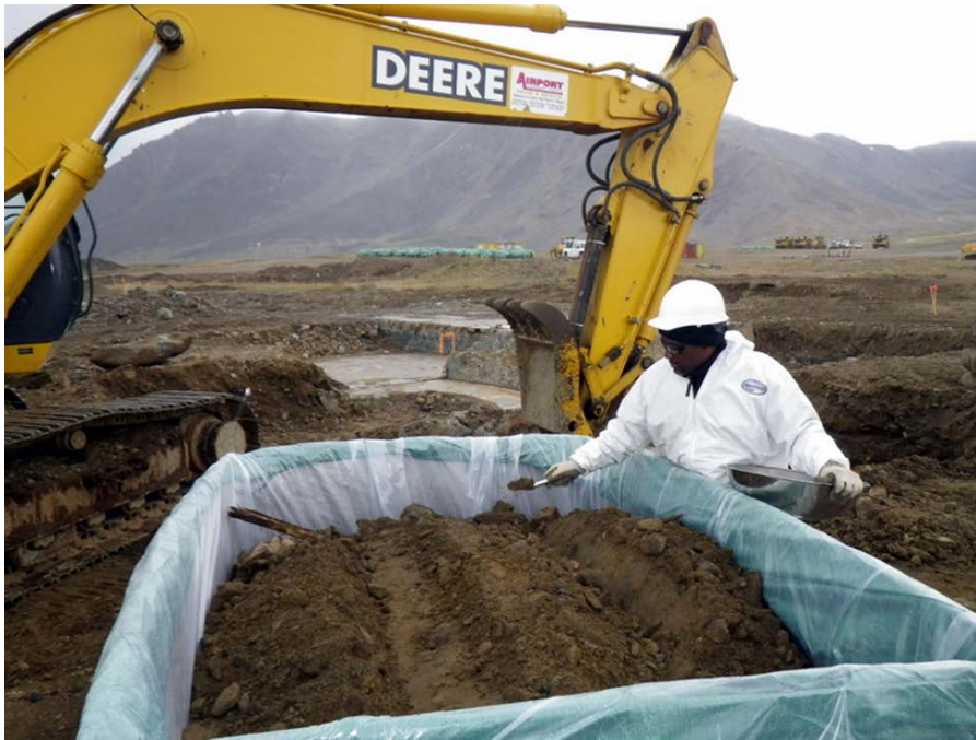
Photograph 35 Collecting samples from bulk bags from Site 13 August 22, 2011
