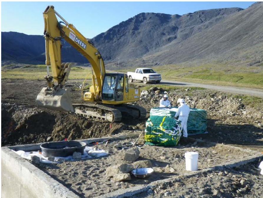
Photograph 46 Excavating and bulk bagging polychlorinated biphenyls- (PCB-) contaminated soil August 18, 2011
