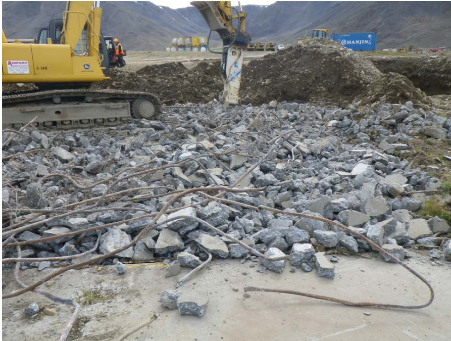
Photograph 19 Breaking up concrete at the MOC August 9, 2011
