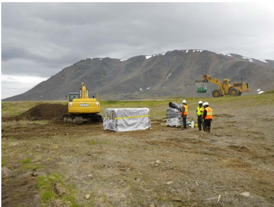
Photograph 1 Bulk bag loading at eastern tank footprint in Main Operations Complex (MOC) July 16, 2011
