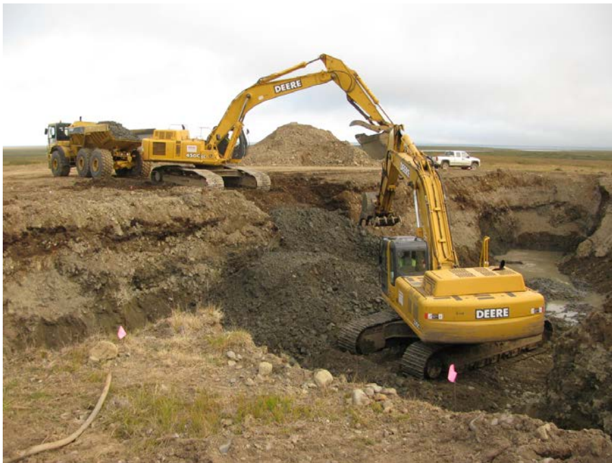
Photograph 16 Excavation of POL-contaminated soil at A1 August 5, 2011
