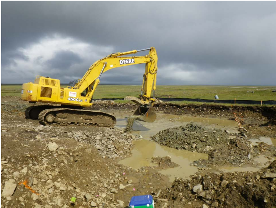
Photograph 15 Removing soil from 2 feet below water at J1A August 3, 2011
