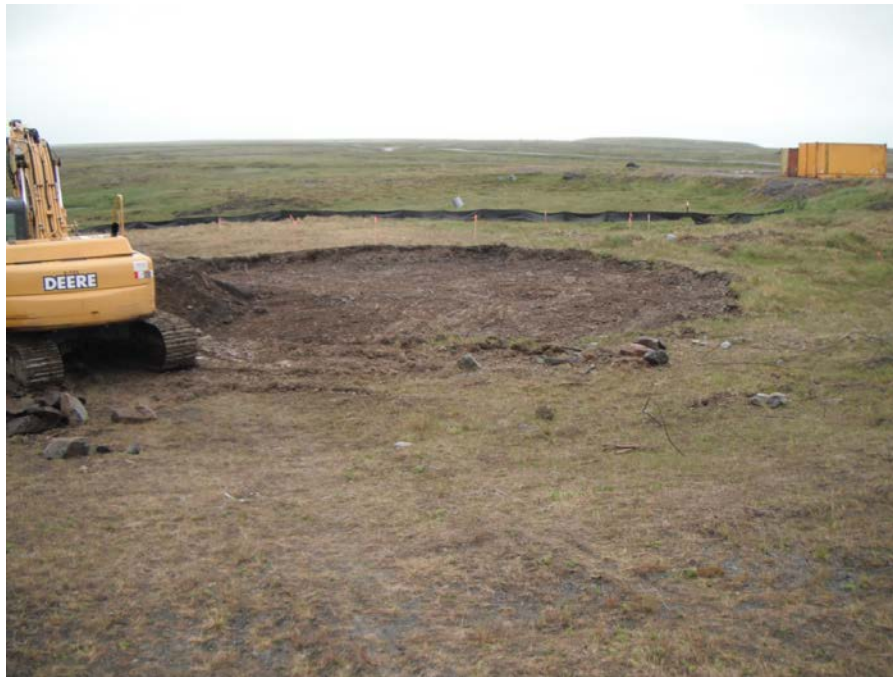
Photograph 3 Excavating eastern tank footprint at the MOC July 18, 2011
