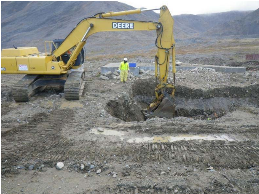
Photograph 48 Sidewall sampling with excavator and sampling attachment September 18, 2011
