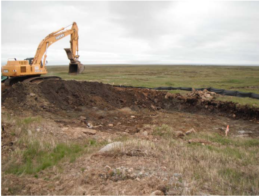
Photograph 9 Excavation of contaminated material 2-4 feet below ground surface (bgs) at J1A July 21, 2011
