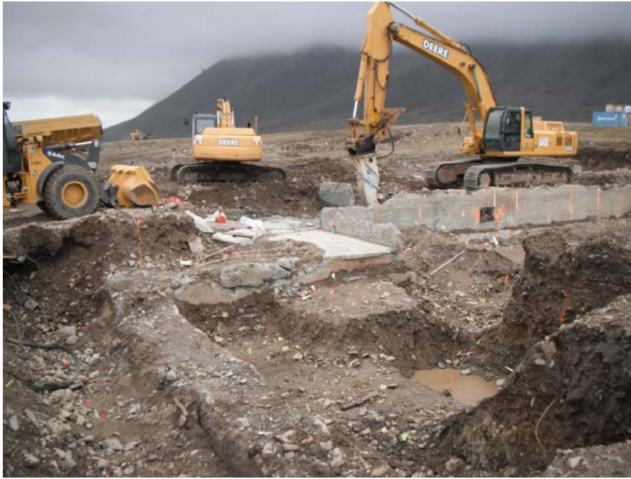
Photograph 37 Concrete removal, material to be used as backfill at A1 excavation September 11, 2011
