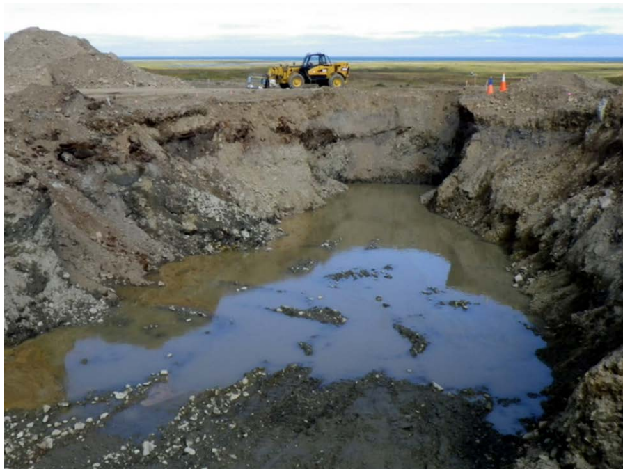
Photograph 22 Groundwater flowing into deepened A1 excavation August 20, 2011
