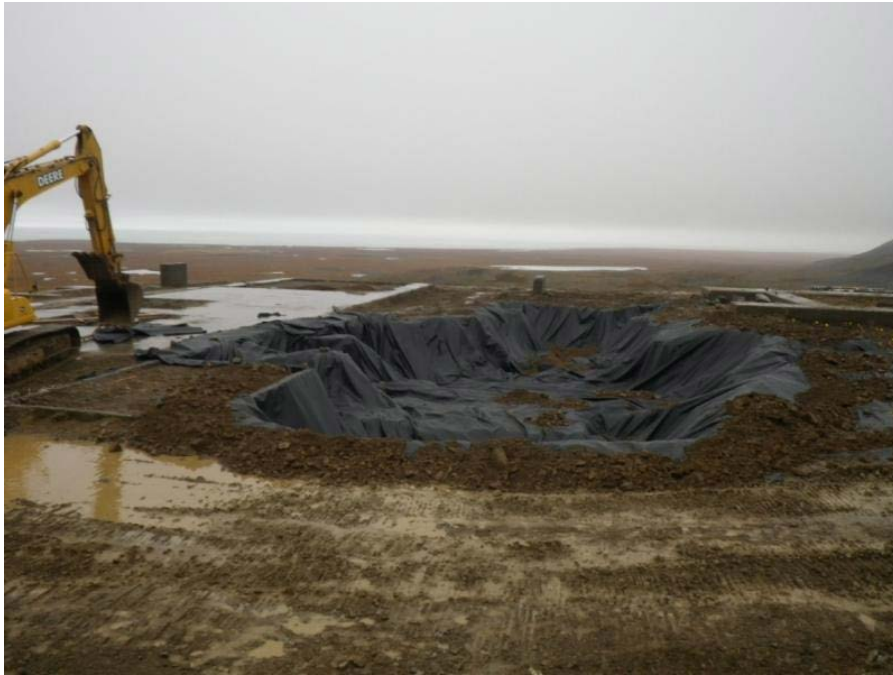
Photograph 49 Placing liner in the Site 31 excavation Northeast Cape September 25, 2011 Direction: Northeast
