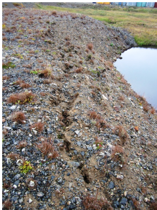
Photo No. 5 – 14 September 2013 Cracking along the border of the runway at Site 1. View facing east.
