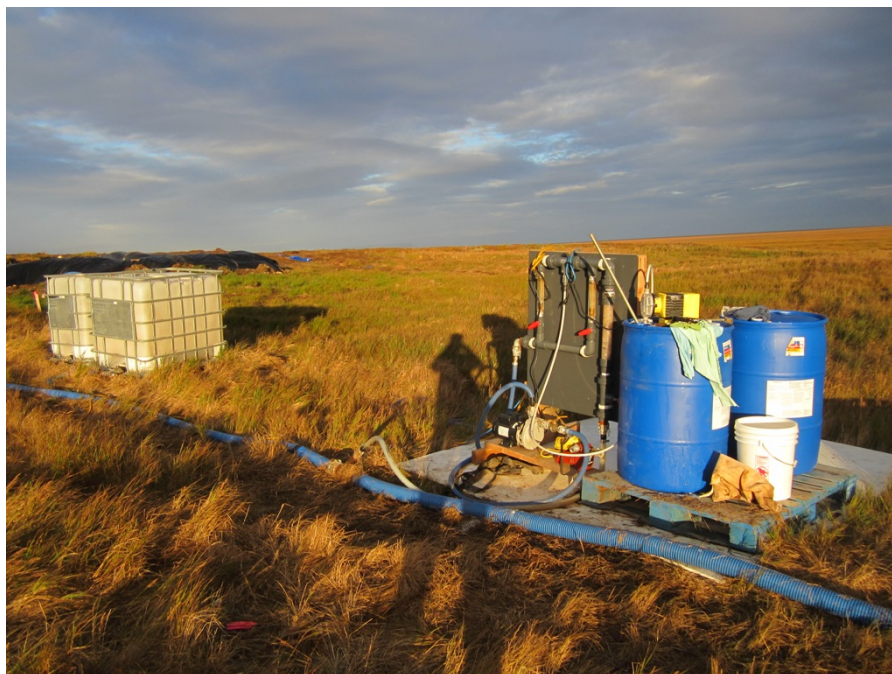
Photo No. 87 – 15 September 2013 Flocculant station for remediation at Site 28. View facing north.
