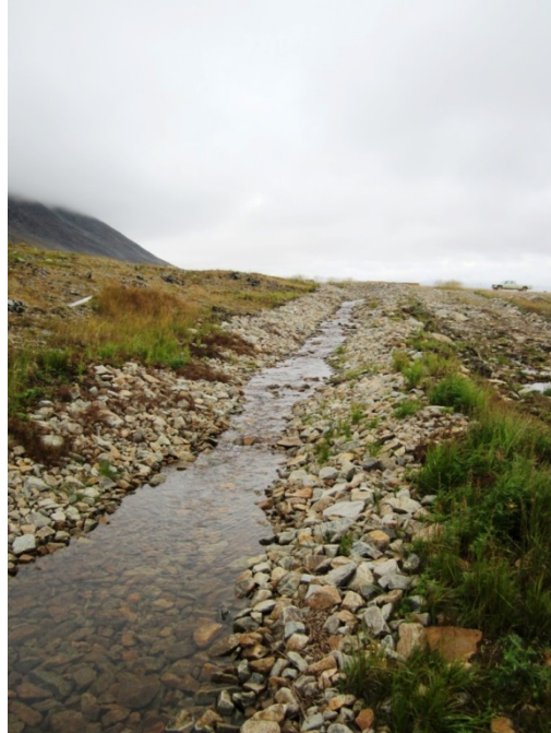
Photo No. 43 – 13 September 2013 Diversion trench adjacent to landfill cap at Site 9. View facing west.
