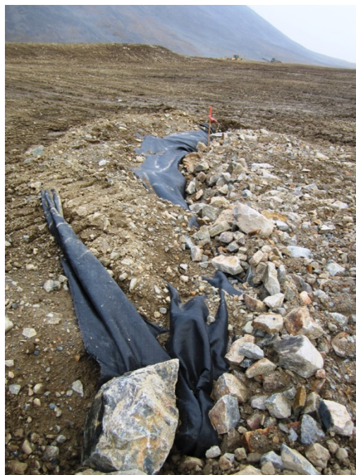
Photo No. 73 – 15 September 2013 Exposed geotextile liner identified at Site 19. View facing west.
