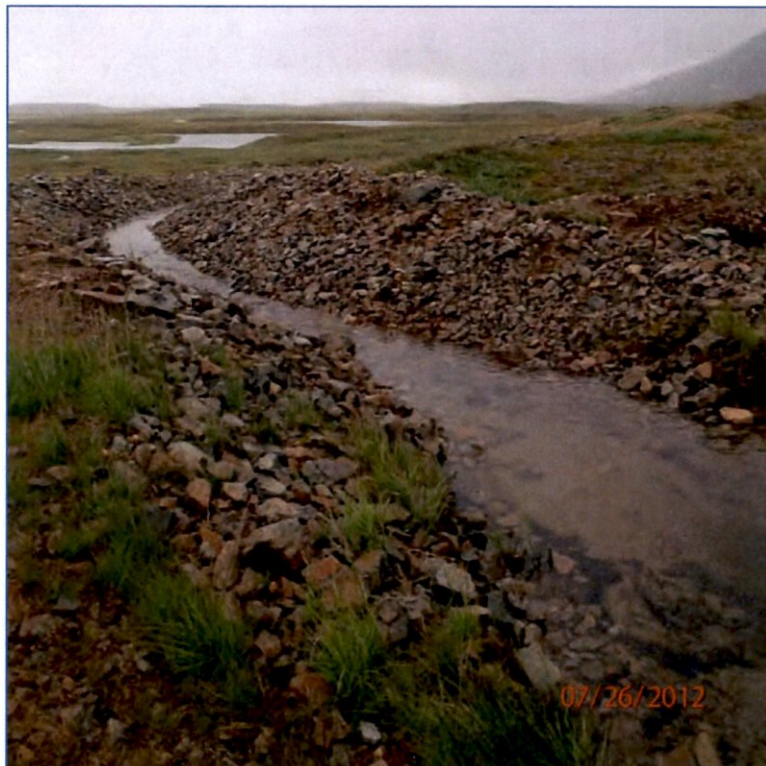
Photo 10: Site 9 Landfill – Pond outlet ditch in good condition and operating efficiently, facing northeast.
