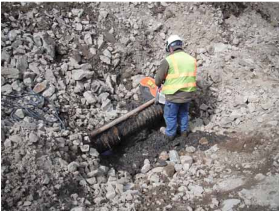
Photograph 32: Site 28 Using chop saw to separate a section of culvert and piping from manhole. Direction: downward view. Date: July 2010.
