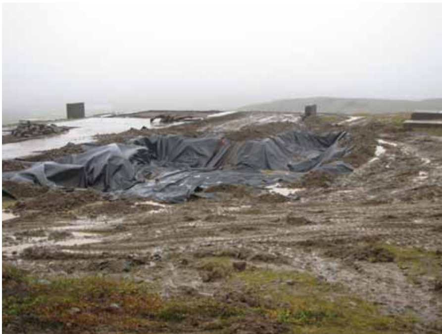
Photograph 42: Site 31 Excavation with liner prior to backfilling. Direction: northeast. Date: September 2010.
