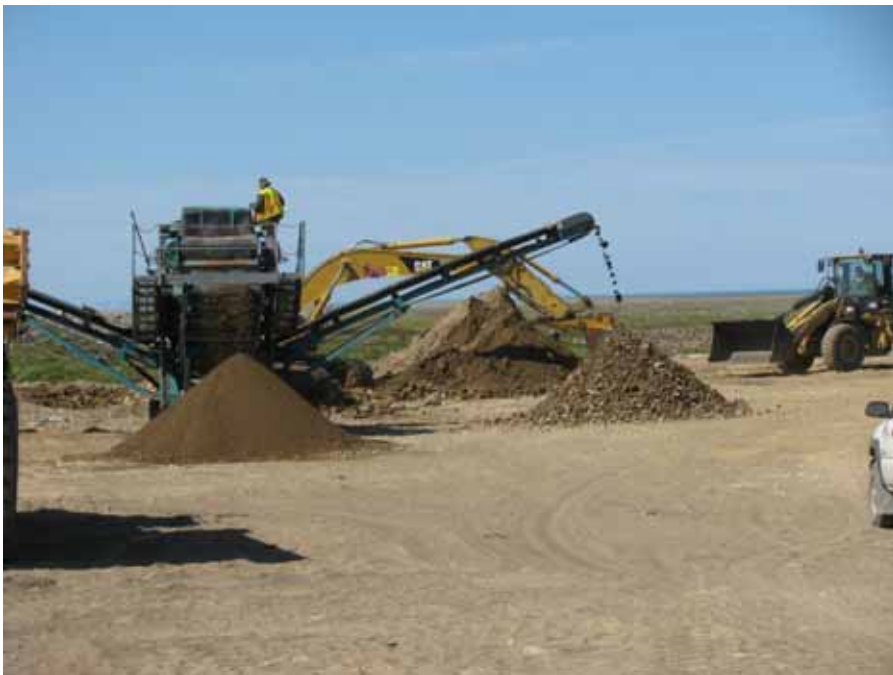
Photograph 52: Rock screen plant in operation at Site 6. Direction: southwest. Date: July 2010.
