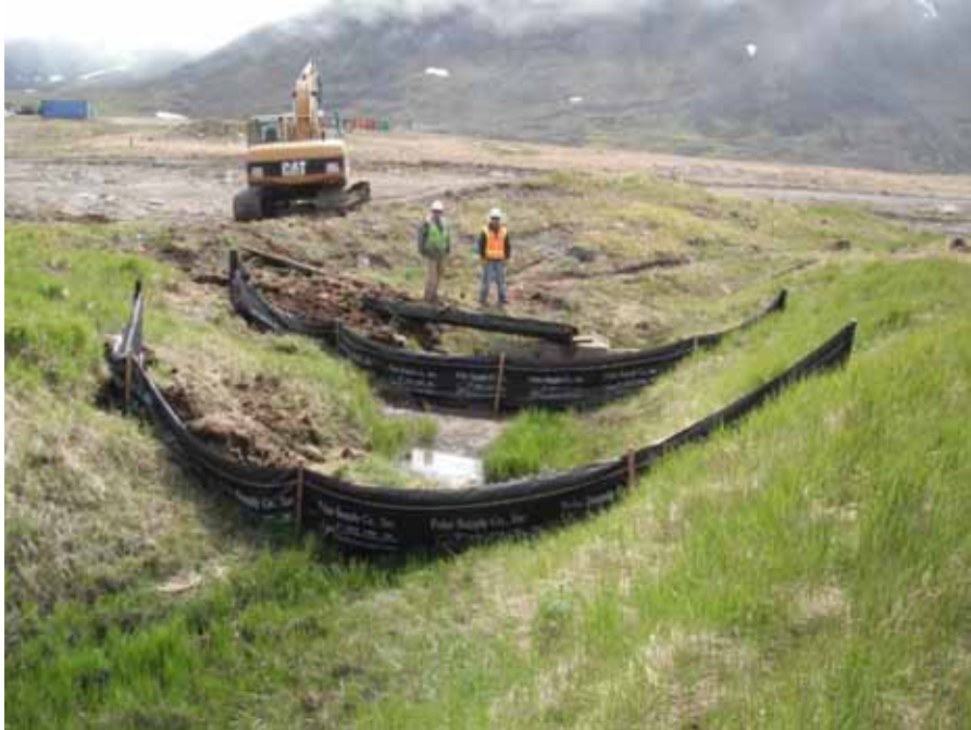
Photograph 35: Site 28 Manhole outfall with silt fences. Direction: southeast. Date: July 2010.
