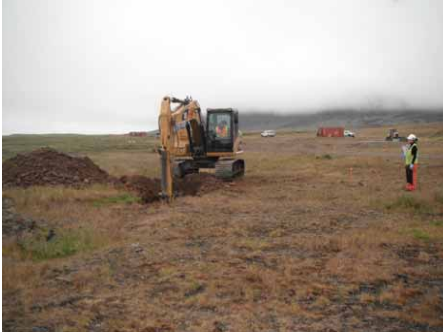
Photograph 49: Test pits being dug at the MOC. Direction: east. Date: August 2010.
