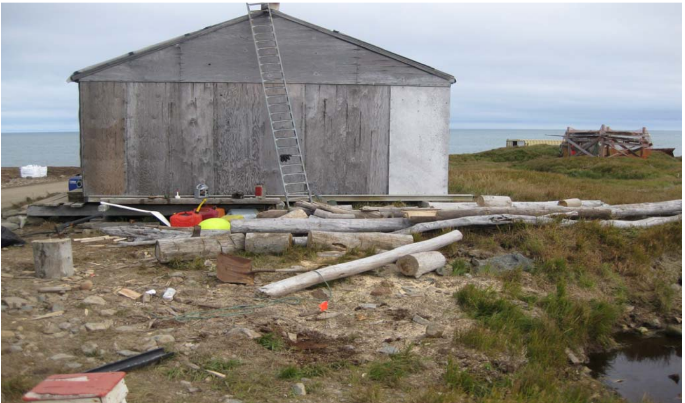
Photograph 28: Soil Sample Location 12NVNCSL28 Collected from Location of Debris Pile #23 Date: September 8, 2012 Direction: North Photographer: L. Nelson
