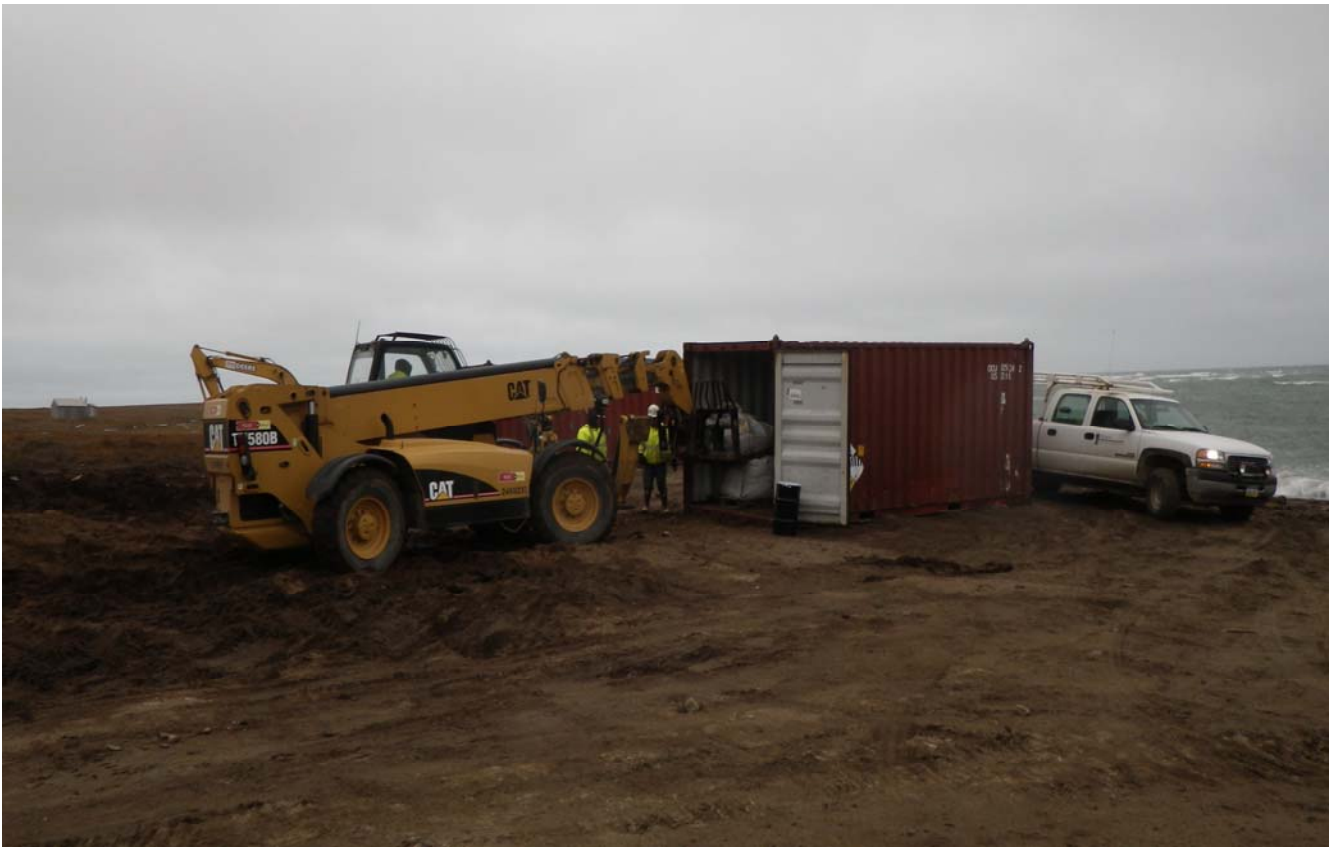
Photograph 21: Loading of CON/HTRW for Transportation and Disposal Direction: Northwest
