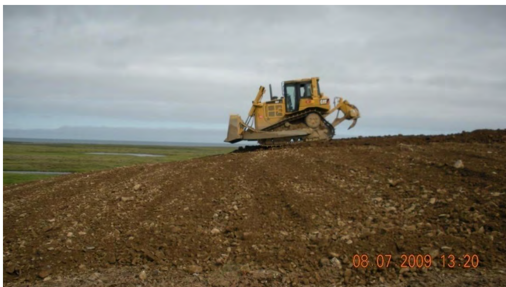
Laying down lifts for landfill cap.
