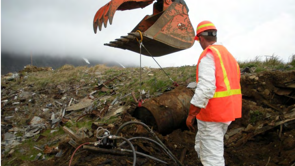
Removing pumped drum with drum lifter and excavator.
