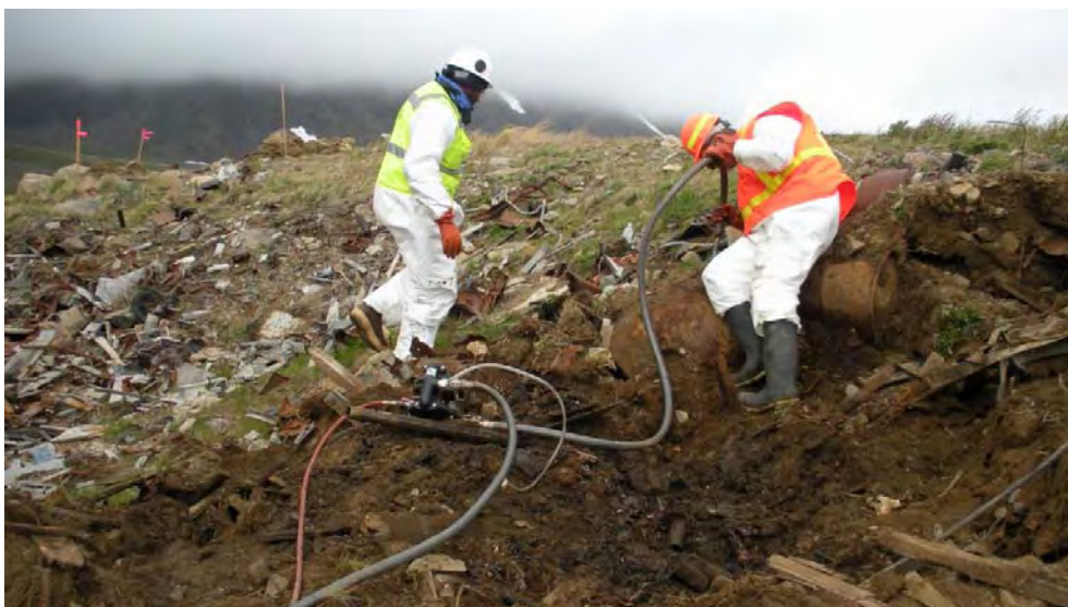
Photograph 3. Field crew pumping liquid out of a corroded drum in the landfill.
