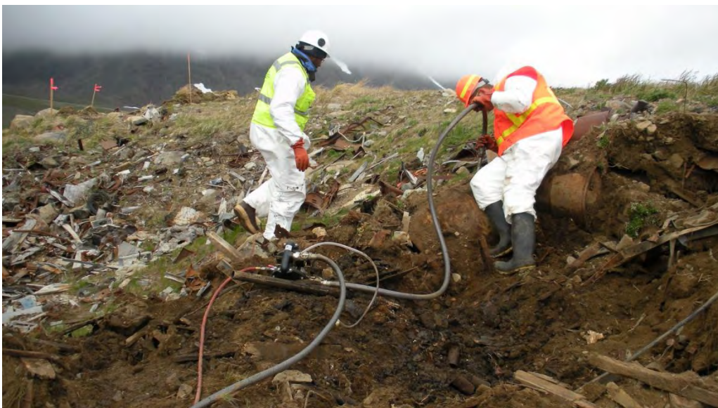
Drum found with oil. In-situ pumping process at landfill.
