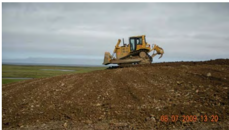
Photograph 5. Laying down and track-walking 6-inch lifts for a minimum of a 24-inch landfill cap.
