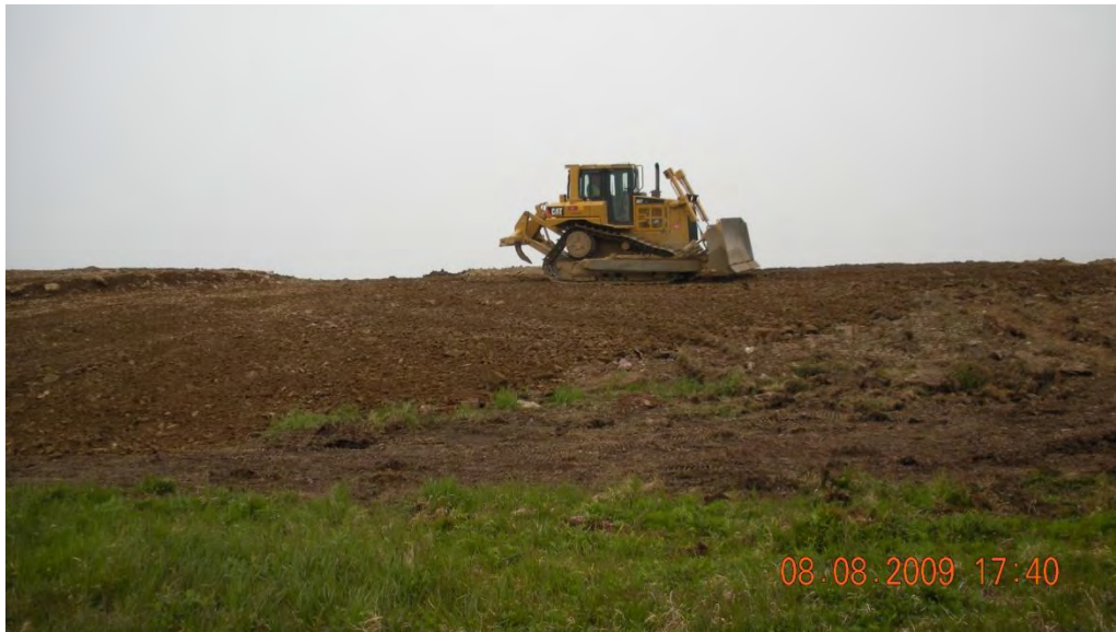
Track walking landfill cap to achieve desired compaction.
