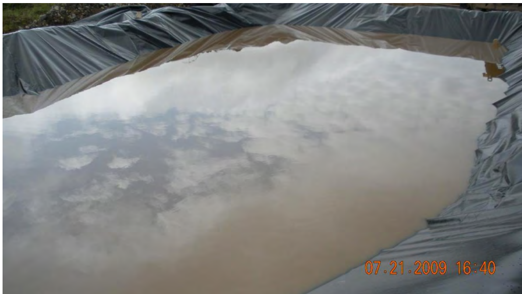
HWAP – Final containment area, post scrubbing, no visible sheen or signs of petroleum contamination.
