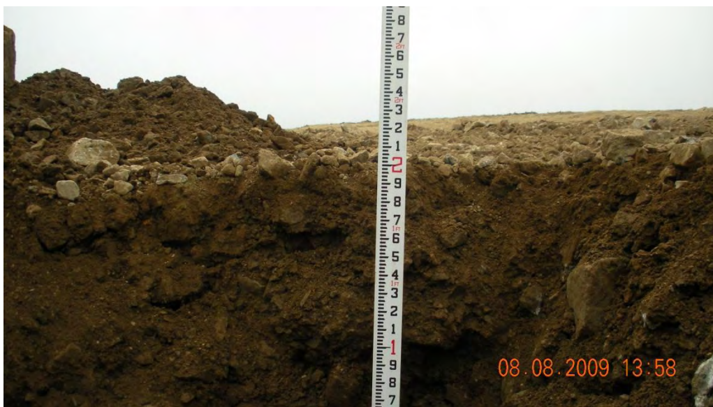
Confirming thickness of landfill cap was at desired thickness of two feet.
