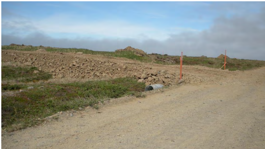
South side of landfill after road around landfill was constructed and culvert placement.
