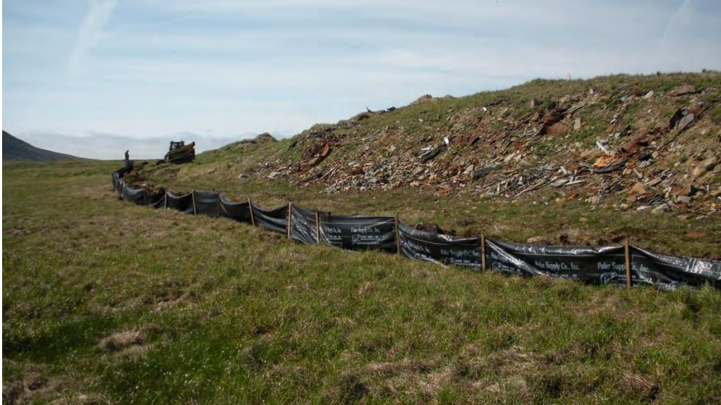
Finished silt fence on southeast slope of landfill, prior to excavation.
