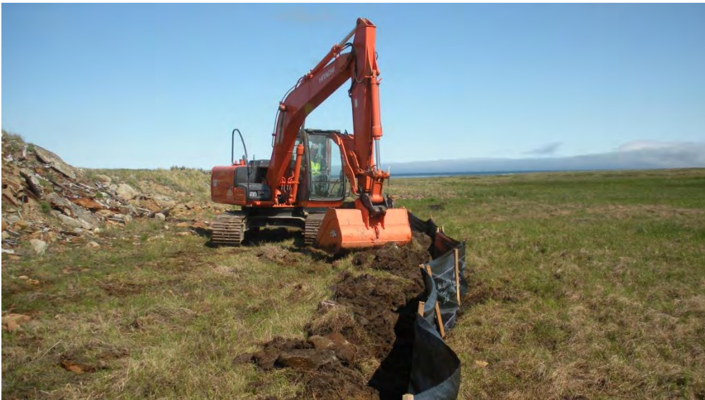
Placing silt fence at toe of slope on southeast slope of landfill.
