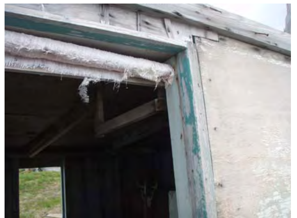
Exterior Door Cloth Building #2 Green LBP door frame
