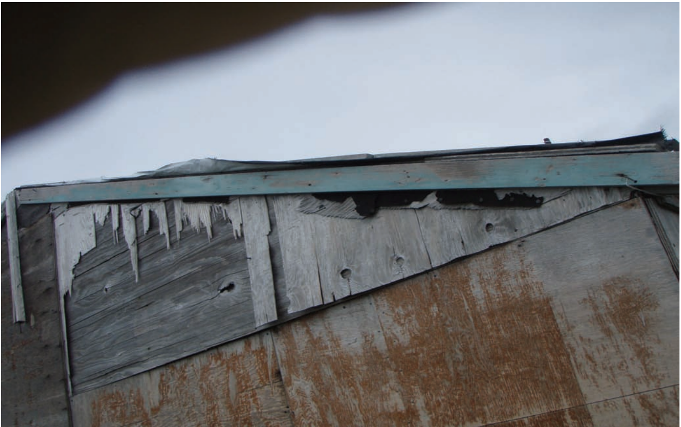
Photograph #13: Structure #3 Green Fascia with LBP Direction: Unknown
