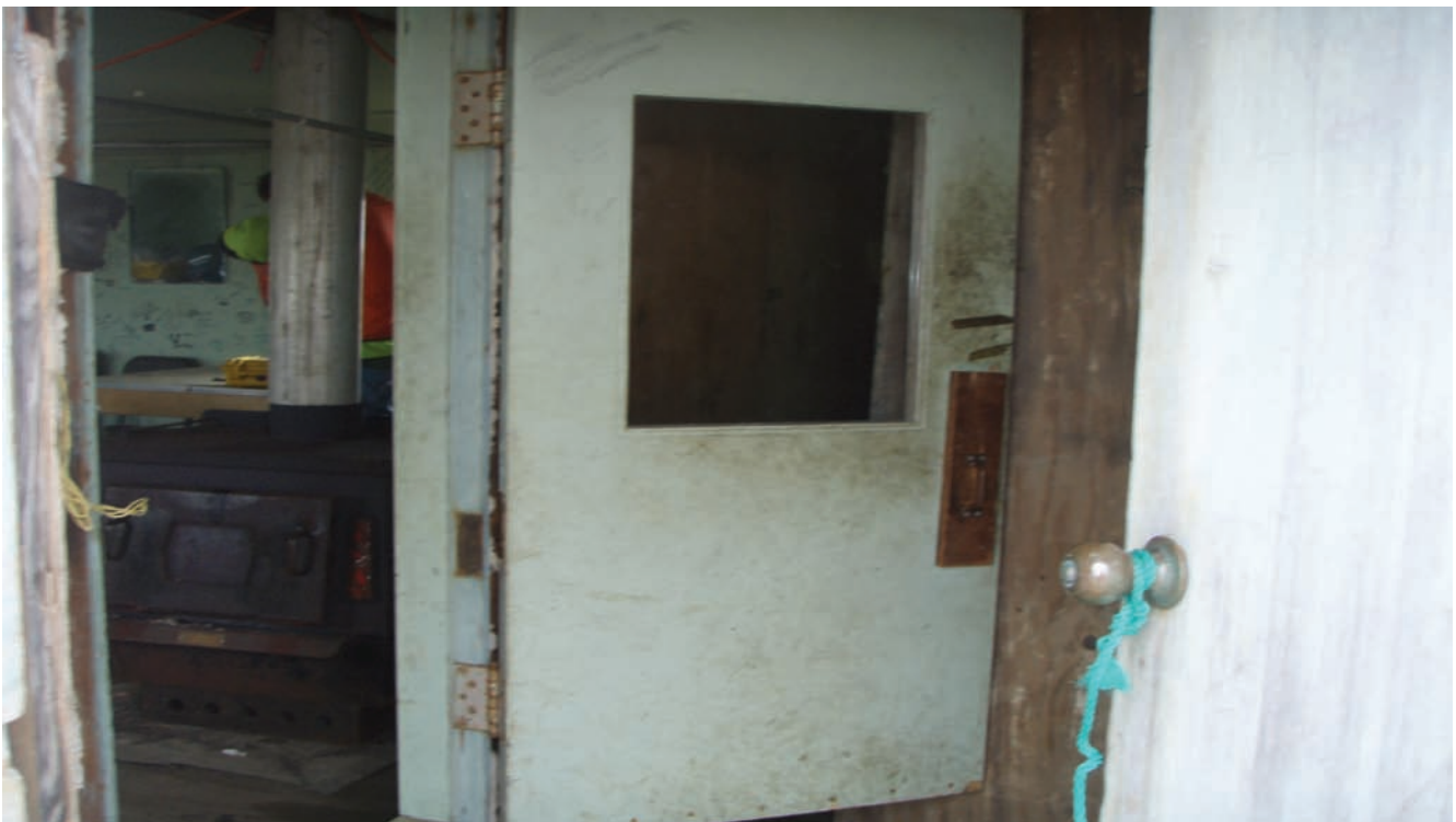
Photograph #2: Structure #1 Interior Door with Green LBP Direction: East
