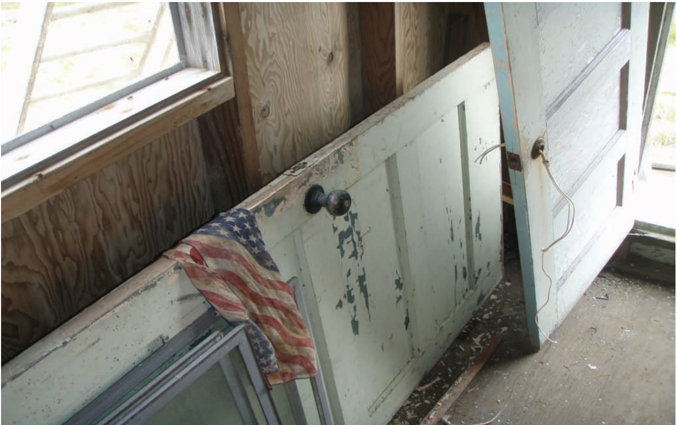
Photograph #37: Structure #11 Interior Door Laying on Ground with LBP Date: July 8, 2009 Direction: Northeast Photographer: T. Ellingboe
