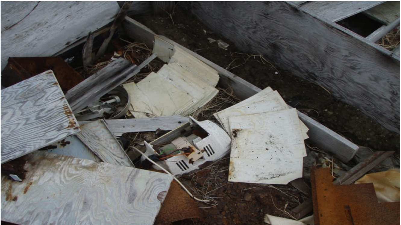
Photograph #34: Structure #9 Exterior with Suspect ACM White Tile Direction: Southeast
