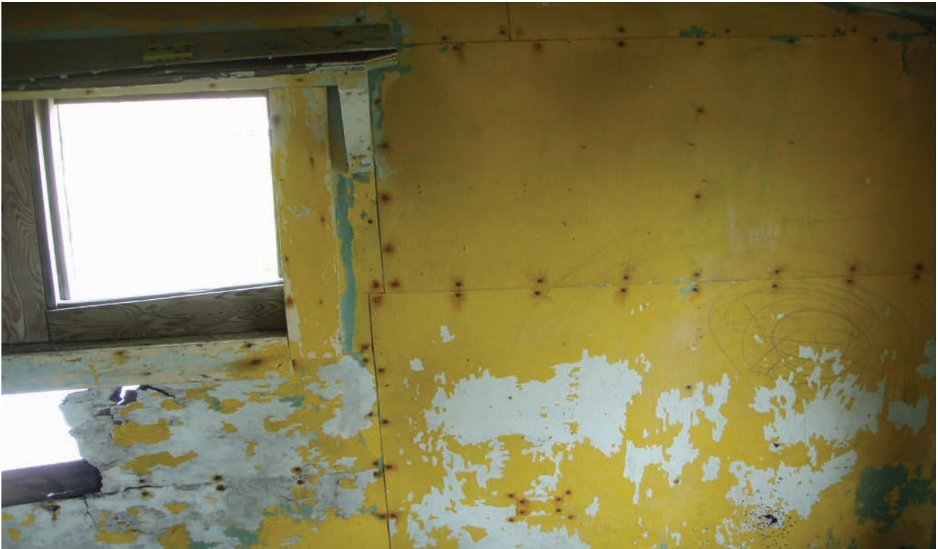
Photograph #18: Structure #6 Interior with Yellow LBP Direction: East
