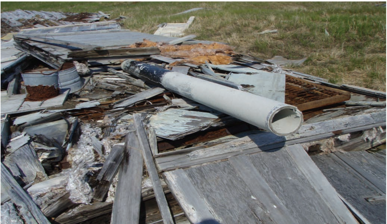
Photograph #4: NVNC Debris Pile with 6" ACM Transite Pipe Direction: West
