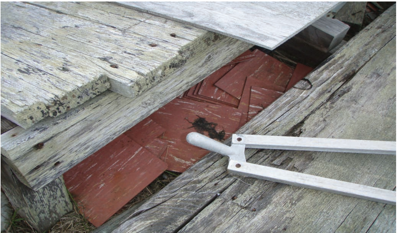
Photograph #10: Intact 9' x 9' ACM Tile Outside Structure #3 Direction: N/A
