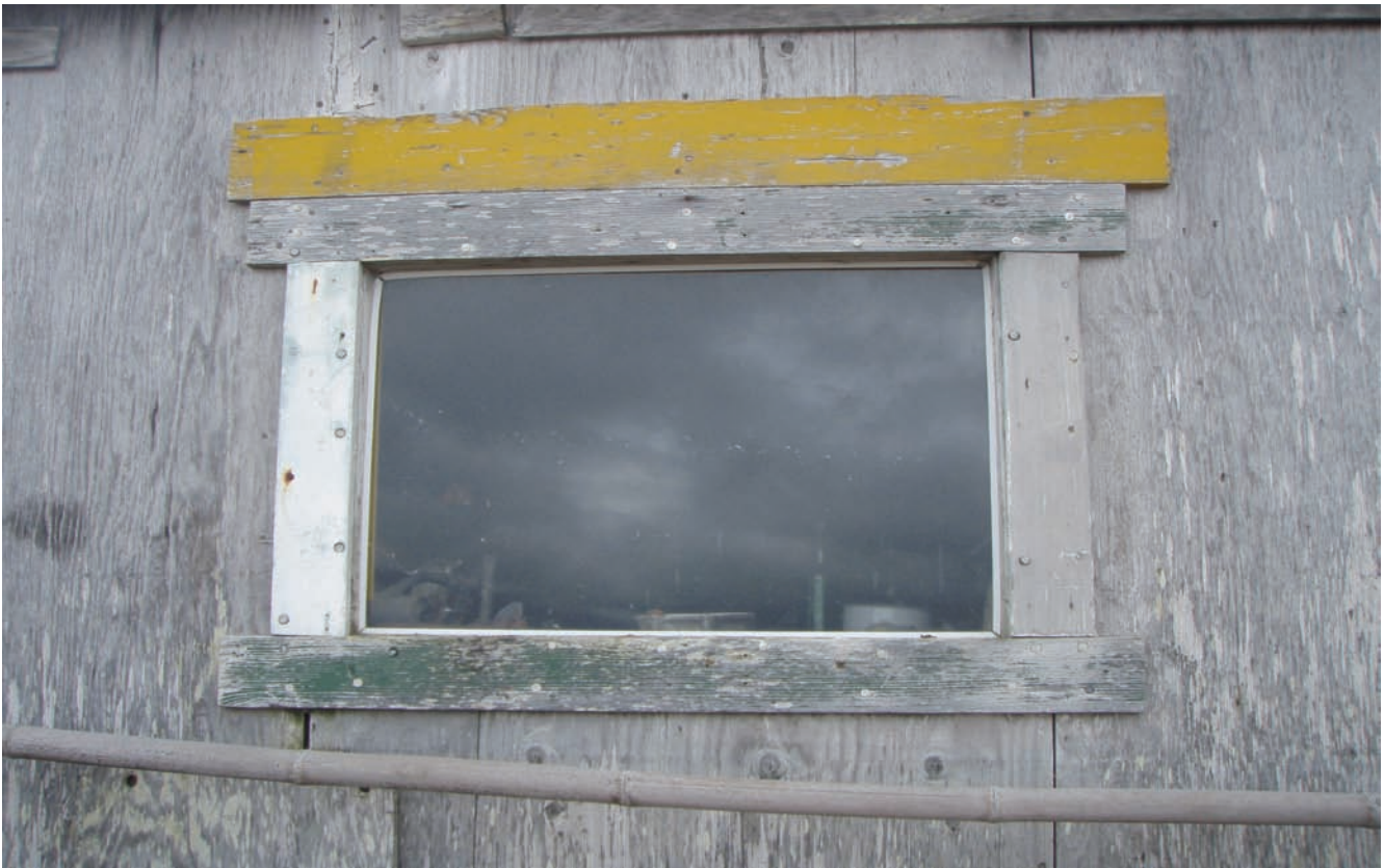
Photograph #11: Structure #3 Window Trim with LBP Direction: South
