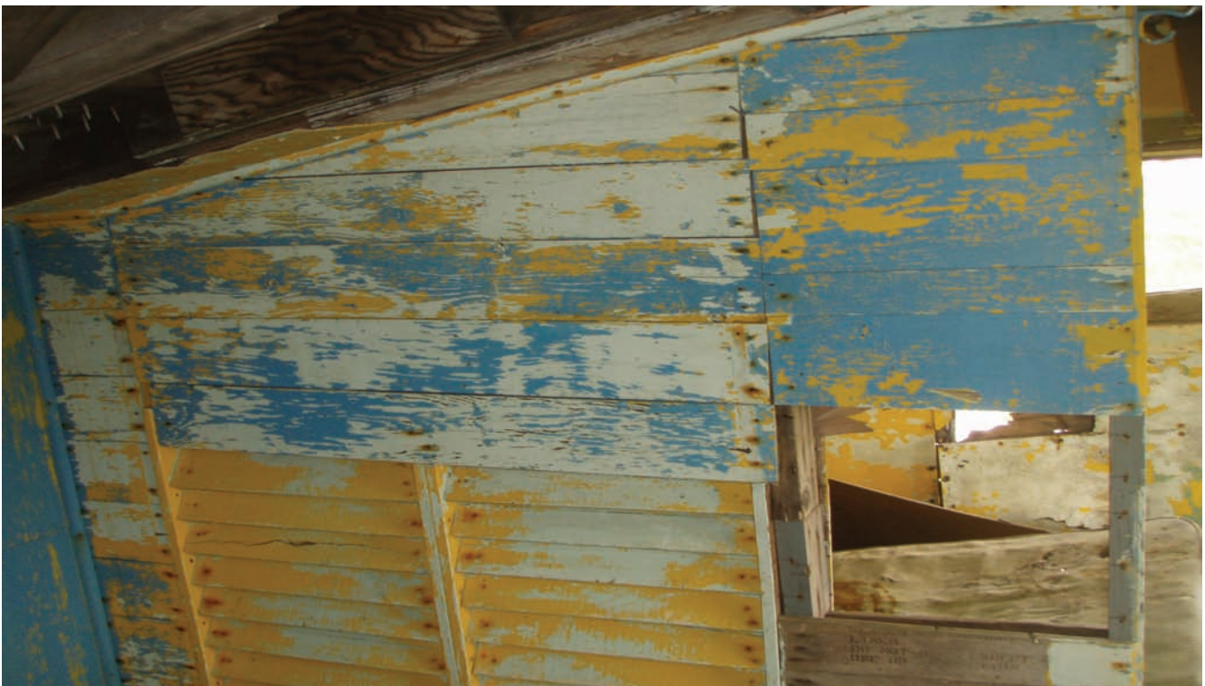
Photograph #20: Structure #6 Interior with LBP Direction: East
