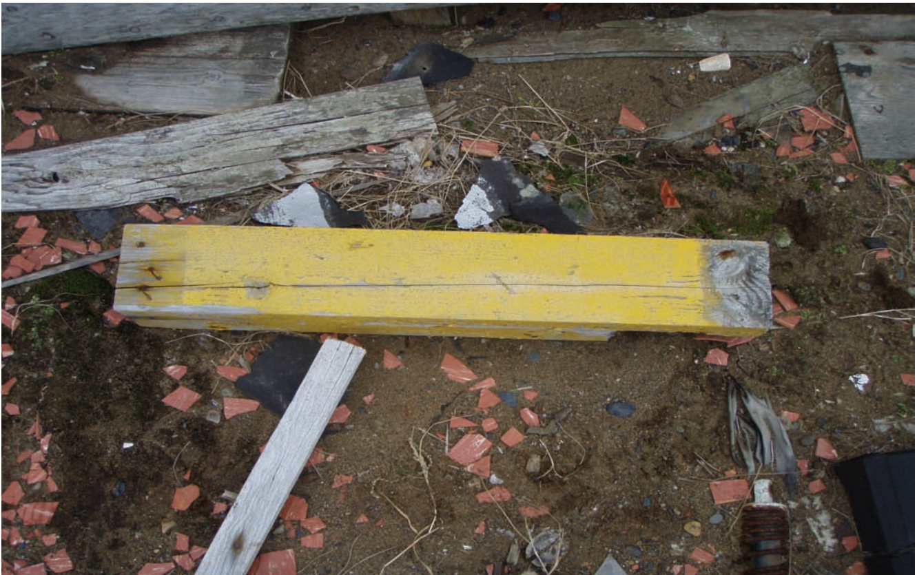
Photograph #19: Structure #5 Exterior 4" x 4" Post with Yellow LBP Direction: South
