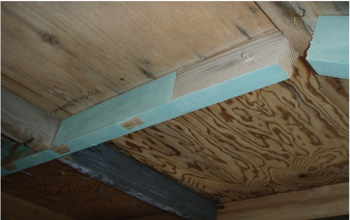
Photograph #21: Structure #7 Interior Roof Joist with LBP Direction: East
