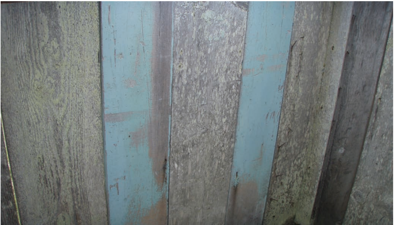
Photograph #50: Structure #12 Interior with Blue LBP Direction: South
