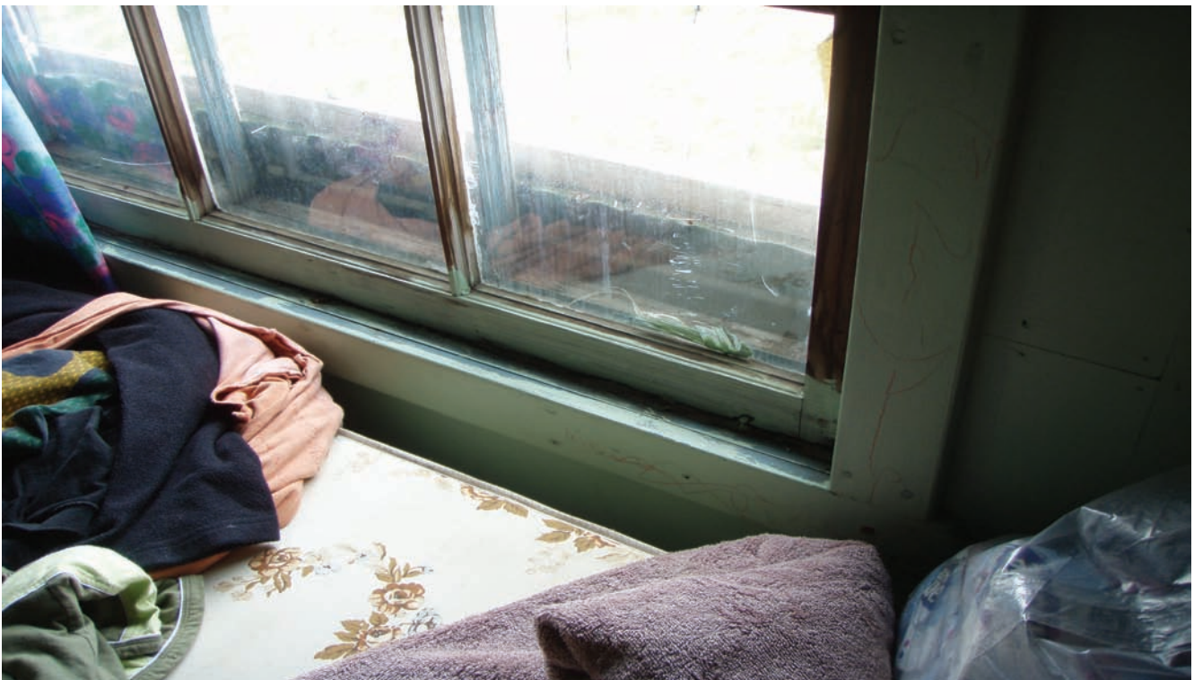
Photograph #32: Structure #3 Green Paint on Window Frame with LBP Direction: West
