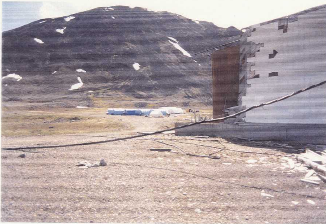
Fig. 3.27 Construction camp site at foot of Kangukhsam Mtn. at Northeast Cape on St. Lawrence Island, Alaska. In foreground is water storage tank in historically wind damaged building. Viewed southerly and photographed on 7/6/94 by Larry Wilkinson, Northwest EnviroService, Inc. on Contract DACA85-93-C00048.
