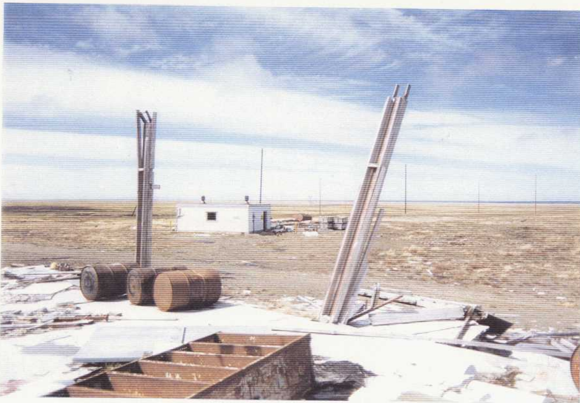
Fig. 3.21 Paint and Dope Storage Building from deck of General Supply Warehouse viewed northeasterly on 7/6/94. Photographed at Northeast Cape, St. Lawrence Island, Alaska by Larry Wilkinson, Northwest EnviroService, Inc. on Contract DACA85-93-C-0048.
