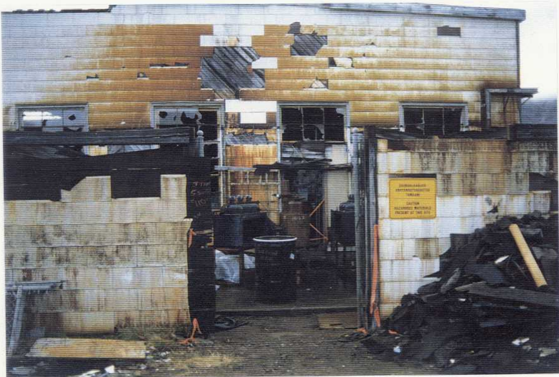
Fig. 3.2 Roof debris removed exposing transformers and switches at Building 110; viewed northeasterly on 7/20/94 at Northeast Cape St. Lawrence Island, Alaska. Photographed by Chuck Heath, Northwest EnviroService, Inc. on Contract DACA85-93-C-0048.
