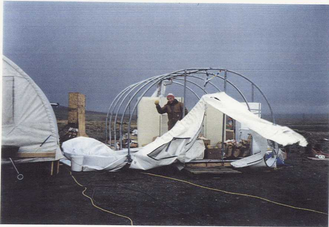
Fig. 3.29 Wind damage to food storage cache following 70 - 90 mph windstorm at construction camp. Viewed westerly on 7/7/94 at Northeast Cape, St. Lawrence Island, Alaska. Photographed by Michael Naquin, Northwest EnviroService, Inc. on Contract DACA85-93-C-0048.
