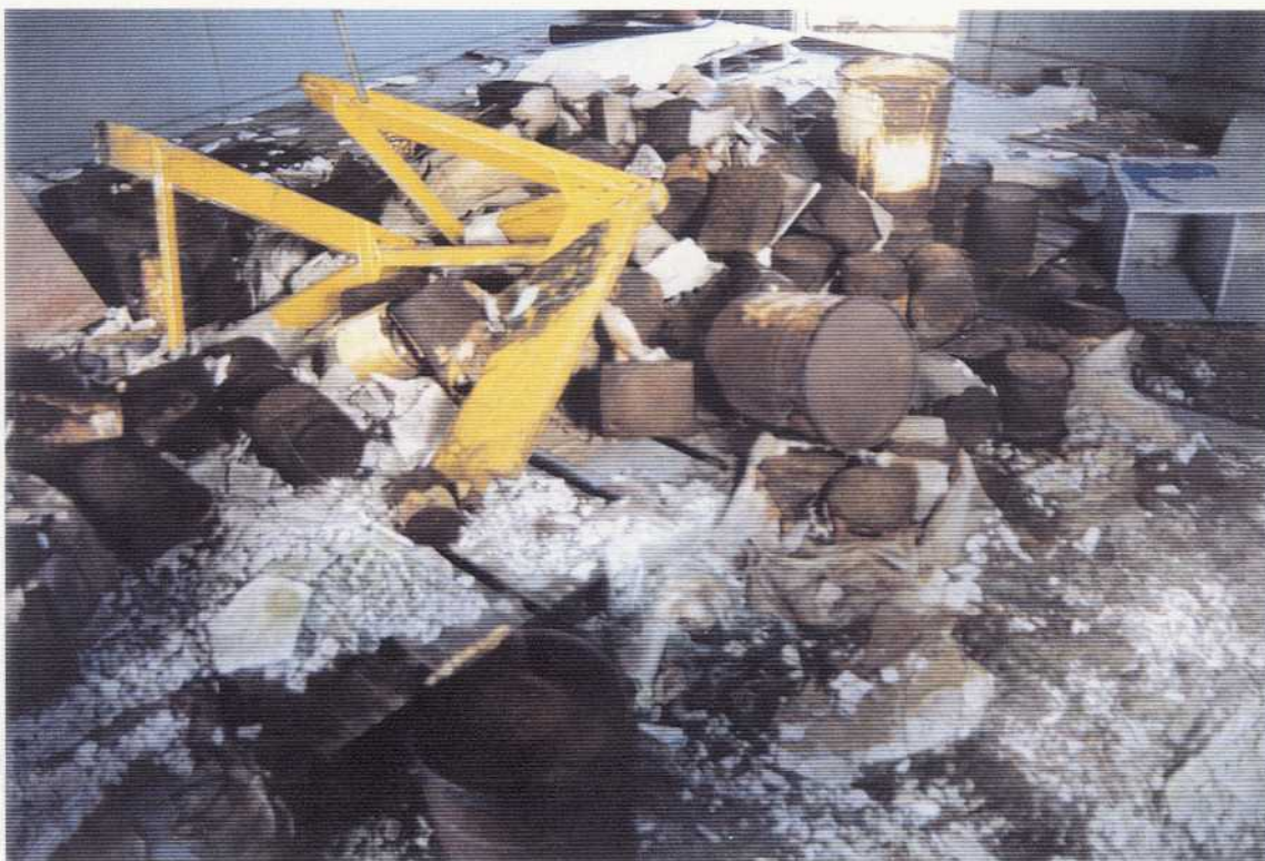
Fig. 3.24 Scattered paint cans and debris inside Paint and Dope Storage Building, viewed northerly on 9/4/93 at Northeast Cape on St. Lawrence Island, Alaska. Photographed by Larry Wilkinson, Northwest EnviroService, Inc. on Contract DACA85-93-C-0048.
