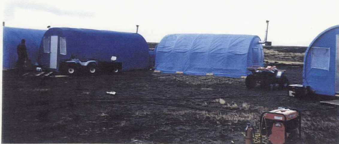
Fig. 3.30 Front end of weather port in pivoted position after 70 - 90 mph windstorm at construction camp. Viewed northerly on 7/7/94 at Northeast Cape, St. Lawrence Island, Alaska. Photographed by Michael Naquin, Northwest EnviroService, Inc. on Contract DACA85-93-C-0048.
