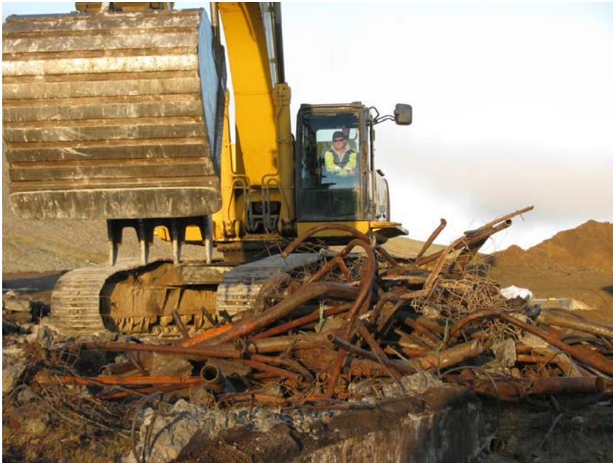
Photograph 70 Metal debris was machine and hand-picked during site work
