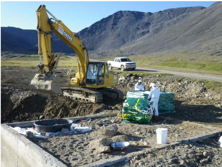
Photograph 46 Excavating and bulk bagging polychlorinated biphenyls- (PCB-) contaminated soil
