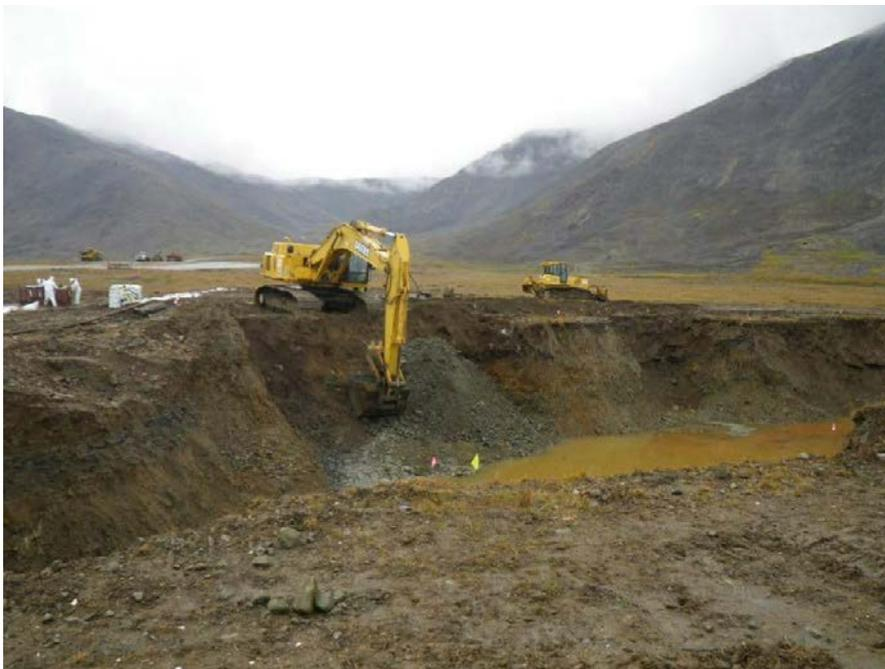
Photograph 24 Excavating POL hot spots Northeast Cape
