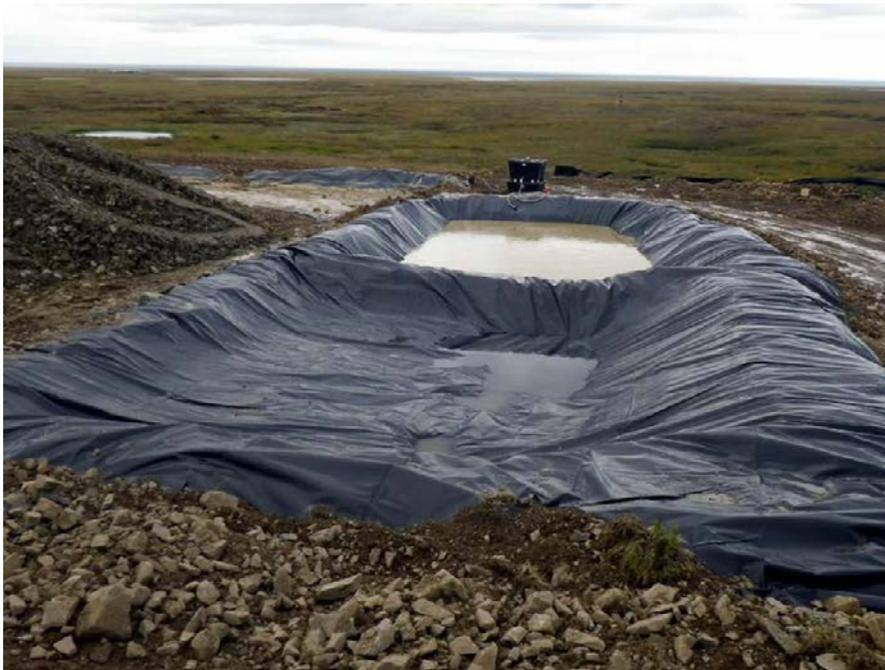
Photograph 23 Lined sumps with filtered water from Northeast Cape
