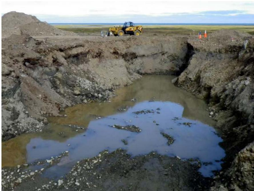
Photograph 22 Groundwater flowing into deepened A1 excavation
