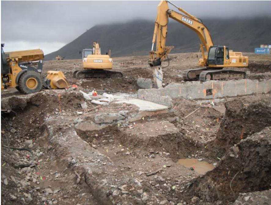
Photograph 37 Concrete removal, material to be used as backfill at A1 excavation
