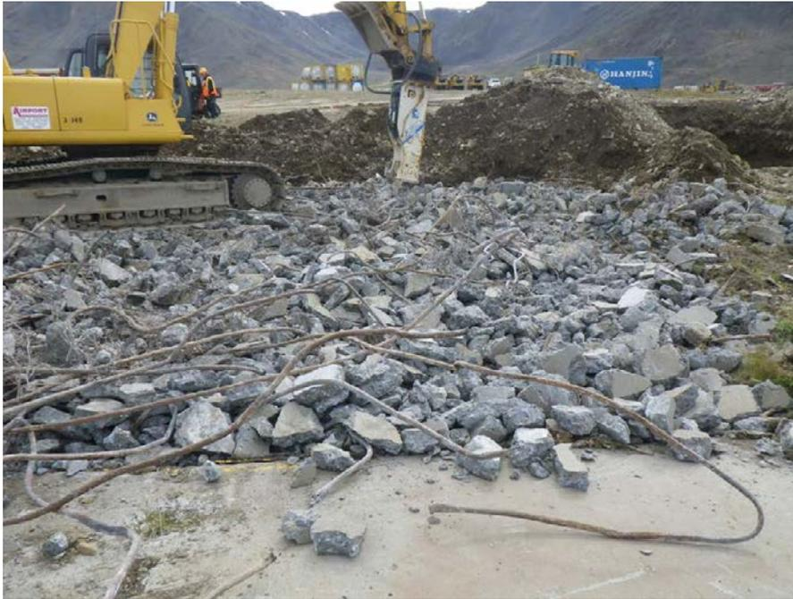
Photograph 19 Breaking up concrete at the MOC
