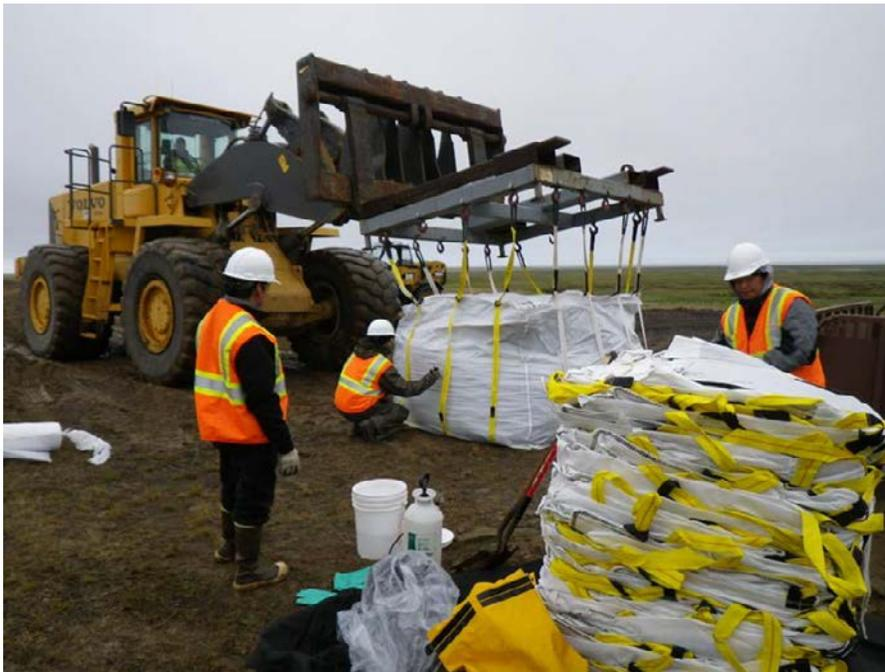
Photograph 2 Bag loading and marking in MOC tank footprint area
