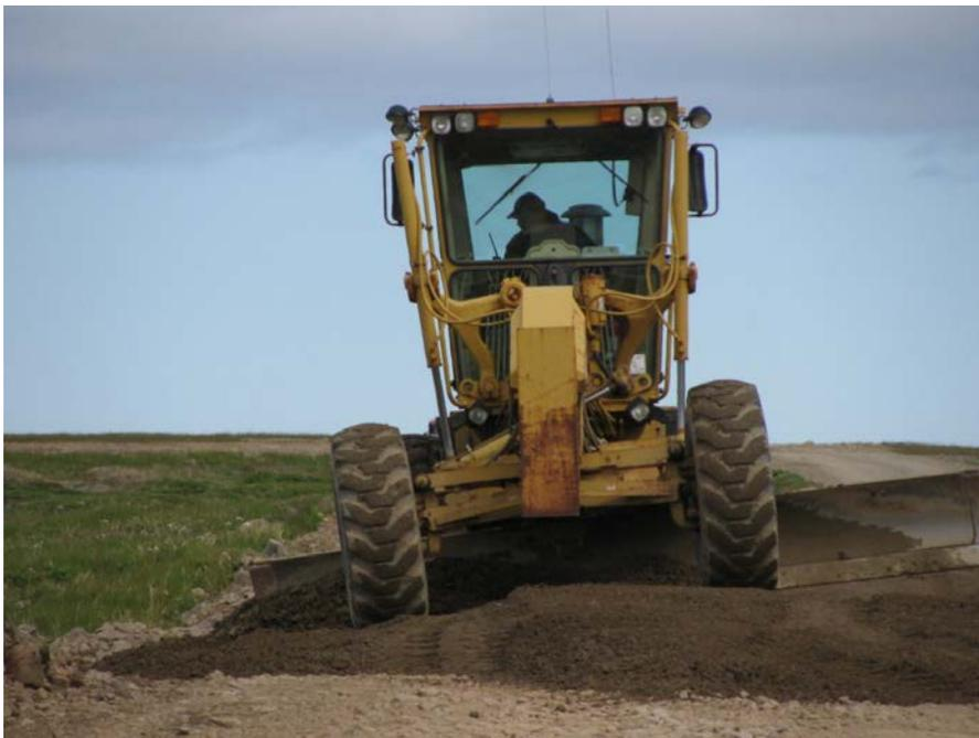
Photograph 74 Road regrading and repair Northeast Cape
