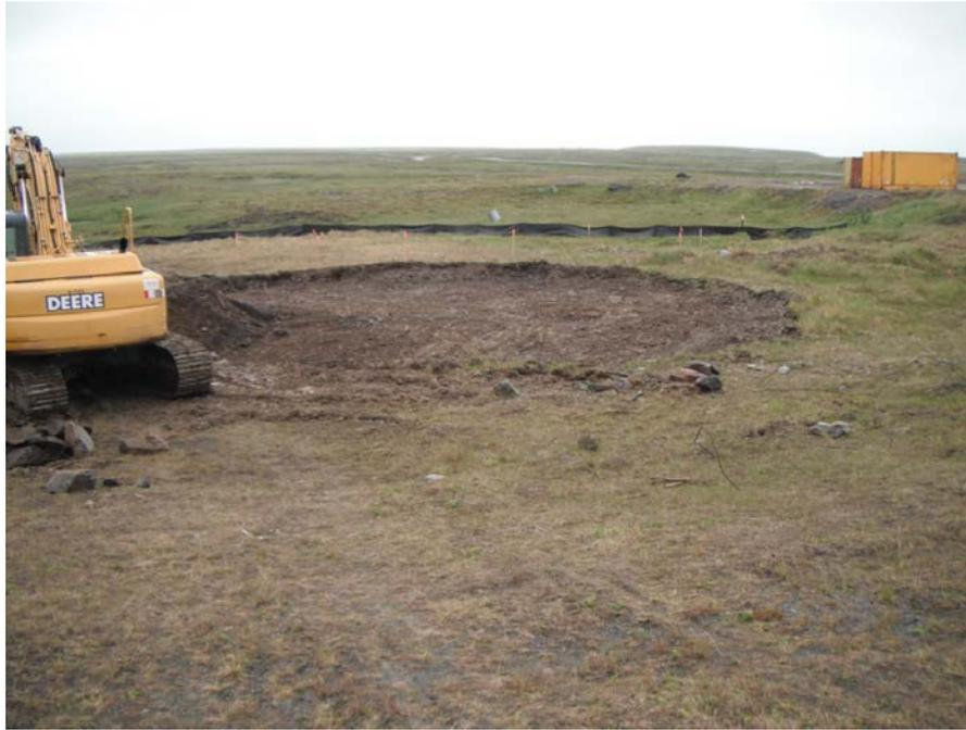
Photograph 3 Excavating eastern tank footprint
