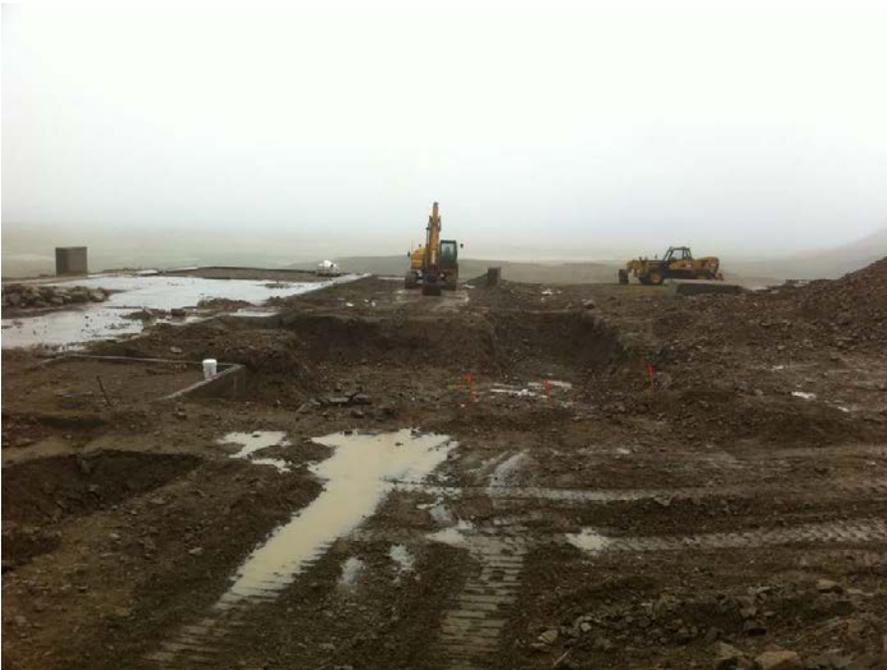
Photograph 44 Water pooling behind berm at Site 31
