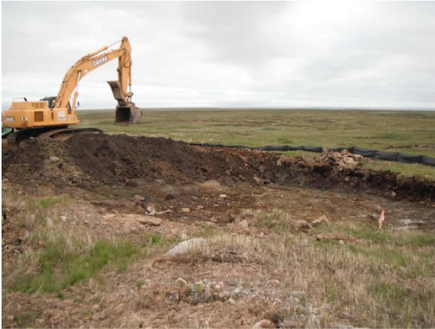
Photograph 9 Excavation of contaminated material
