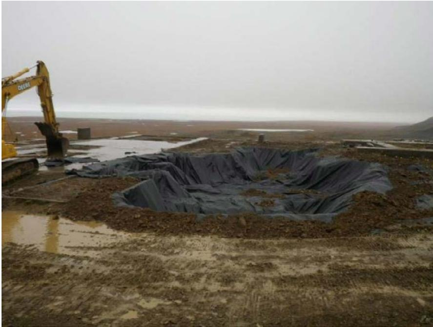
Photograph 49 Placing liner in the Site 31 excavation Northeast Cape
