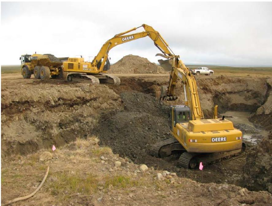
Photograph 16 Excavation of POL-contaminated
