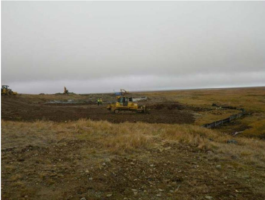
Photograph 25 Backfilling the J1A excavation
