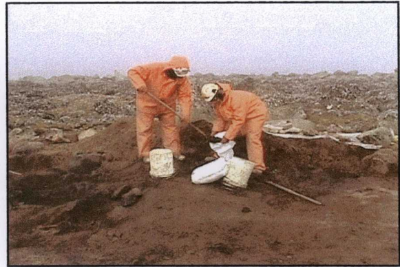
Photo 20: Shovels used to excavate contaminated soil at Site 4/Area 4B.
