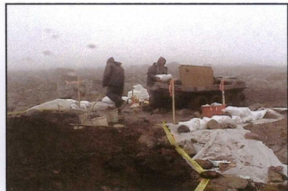
Photo 22: Sand bags filled with soil placed in Argo for transportation down the mountain.
