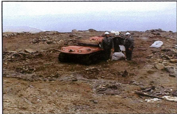
Photo 15: Workers loading bags containing small pieces of metal debris into Argo at Site 4/Area 4A.
