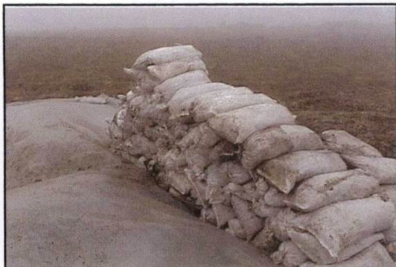
Photo 21: Sand bags filled with contaminated soil at Site 4/Area 4B.
