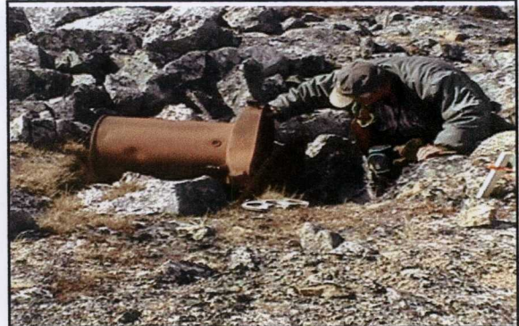
Photo 14: Empty transformer at Site 4/Area 4A.
