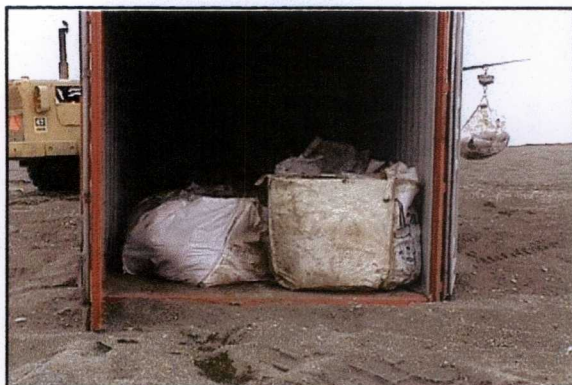
Photo 23: Supersacks filled with contaminated soil placed in connex.
