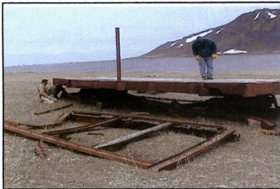
Photo 33: Workers dismantle metal sled at Site 8.
