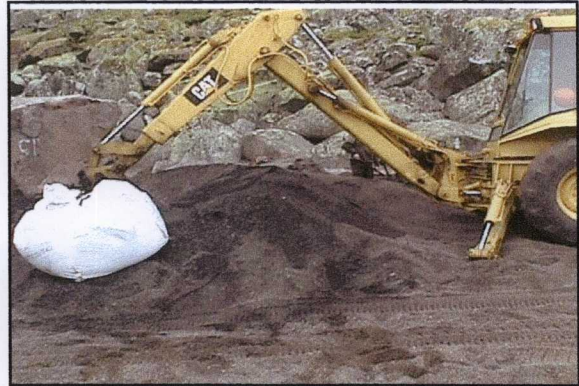
Photo 8: Backhoe moving supersack filled with stained soil at Site 2.
