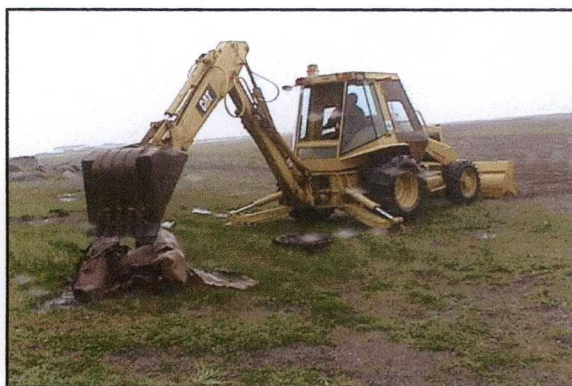
Photo 11: Backhoe preparing to remove empty fuel tank at Site 3.
