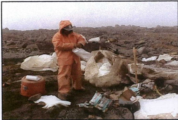
Photo 19: Worker preparing for debris removal at Site 4/Area 4B.
