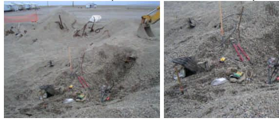
Photo 35: Excavation 18A, severed power line Photo 36: Excavation 18A, severed power line
