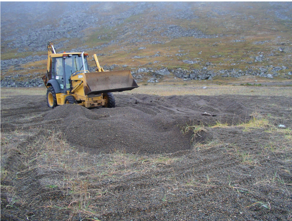
Photo 13: Backhoe filling in exploratory pits near Sevuokuk Mountain. View east.
