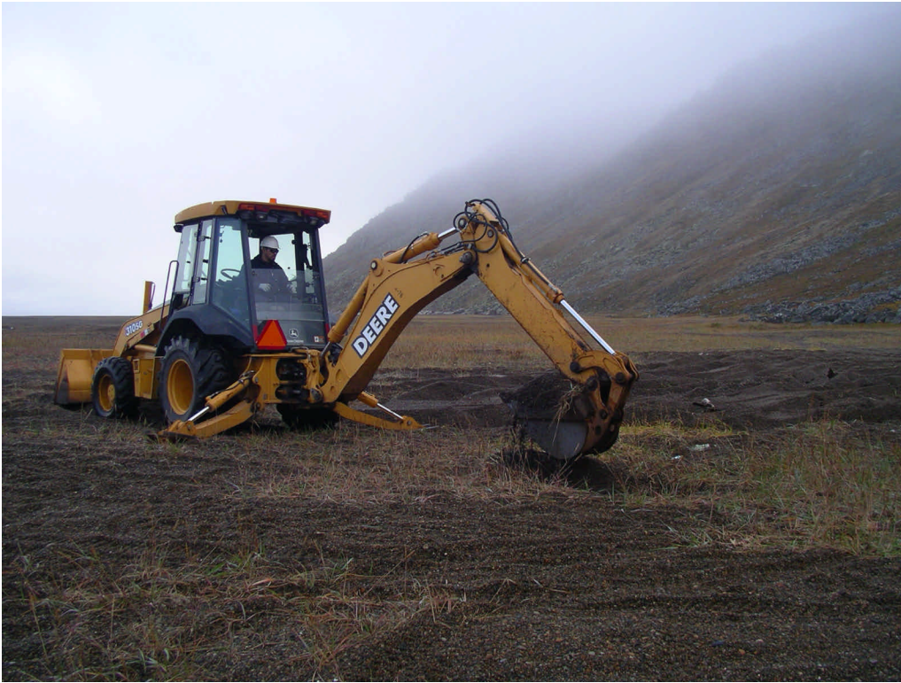
Photo 17: Backhoe digging pits. View north.
