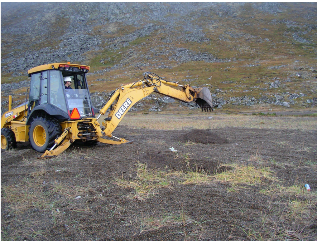
Photo 4: Excavating exploratory pits near base of Sevuokuk Mountain. View east.
