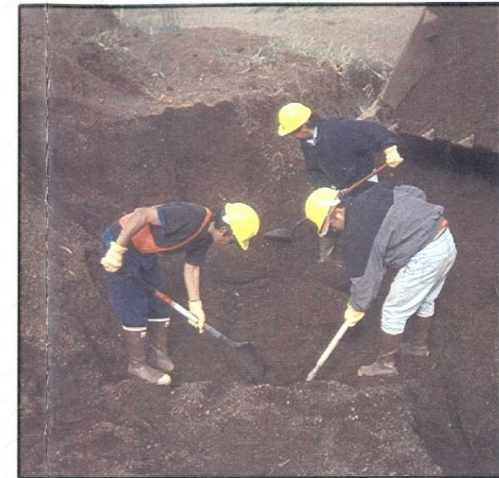
2. MANUAL DIGGING TO EXPOSE DEBRIS
