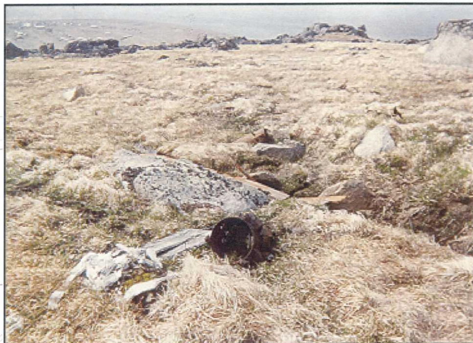
1. FORMER LOCATION OF TRANSFORMERS ON SEVUOKUK MTN.
