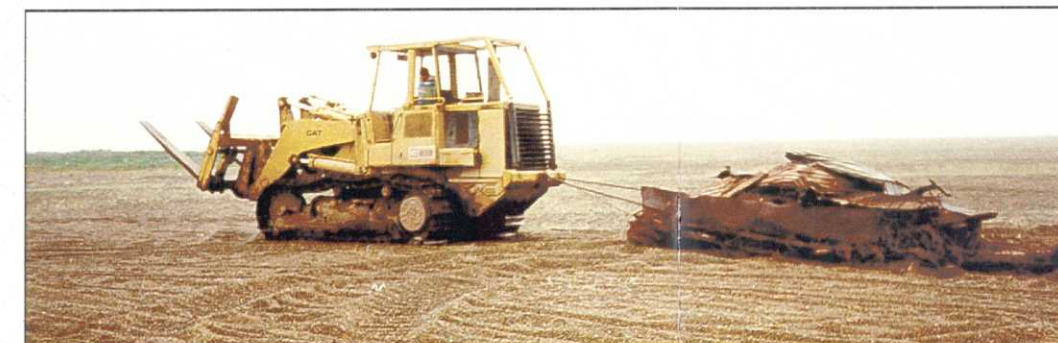
7. TRANSFER OF DEBRIS TO BARGE LANDING AREA FOR DISPOSAL
