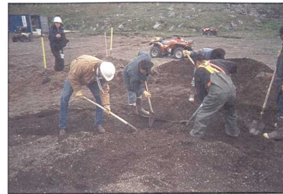
2. MANUAL DIGGING TO EXPOSE DEBRIS
