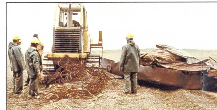
6. TEMPORARY STOCKPILING OF DEBRIS
